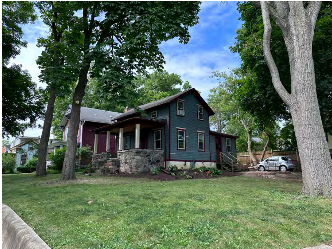
Existing view from northeast
