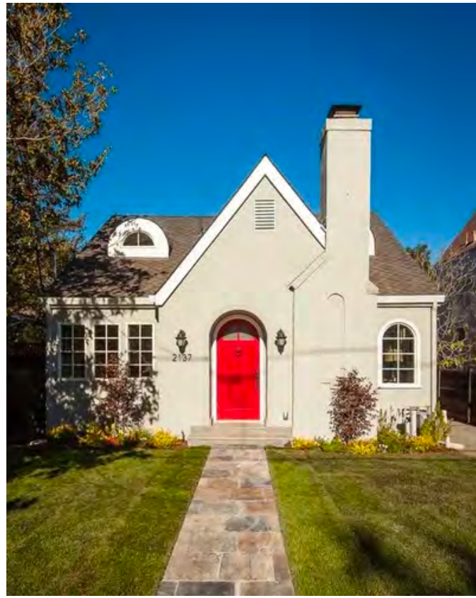
Properly applied synthetic stucco can be seamless, providing a high quality and durable finish that is complimentary to a broad range of architectural styles
