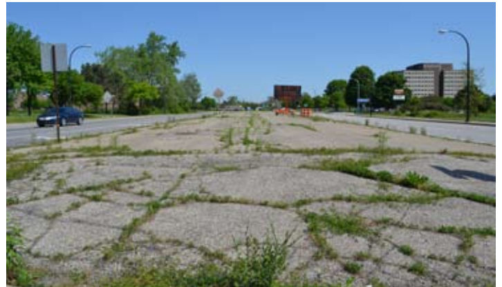
Concrete medians dominate the landscape in Area 2
