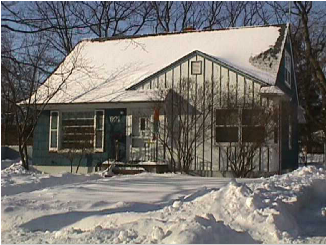
921 DUNCAN ST - 2ND NEIGHBOR TO NORTH
