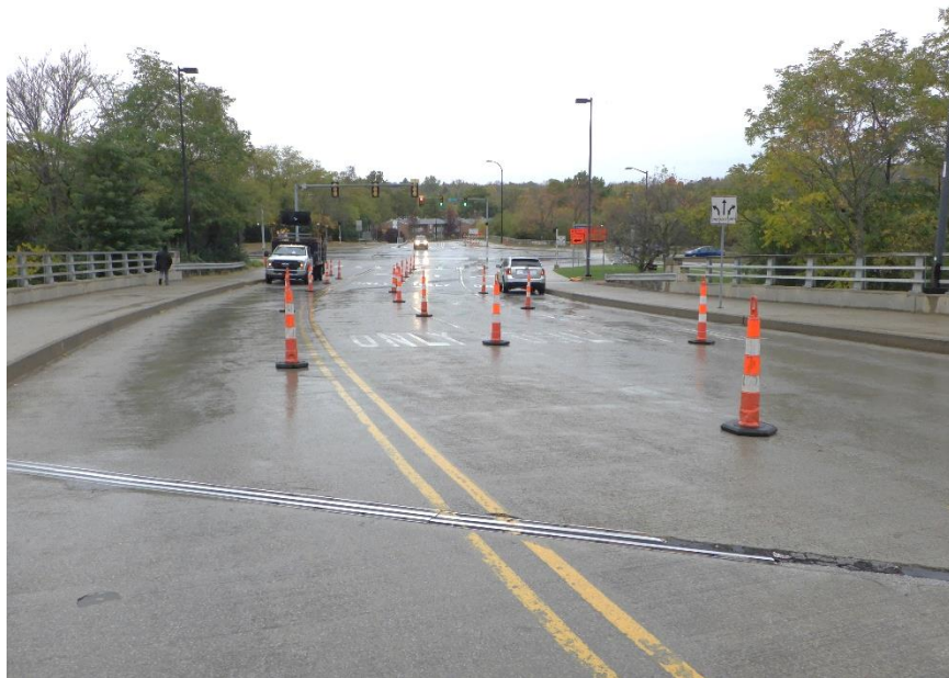
Photograph No. 4 View of Deck Looking North
