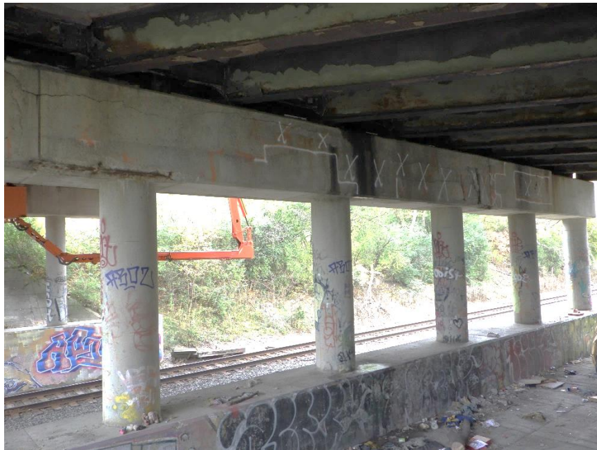
Photograph No. 20 East Portion of North Side of North Pier (Pier 2)
