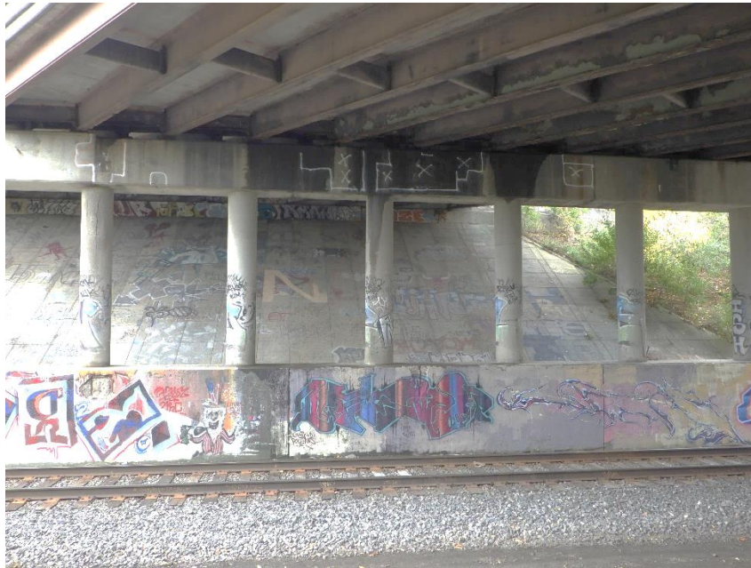
Photograph No. 23 North Side of South Pier (Pier 1)
