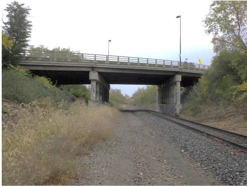
Photograph No. 1 West Elevation Looking East
