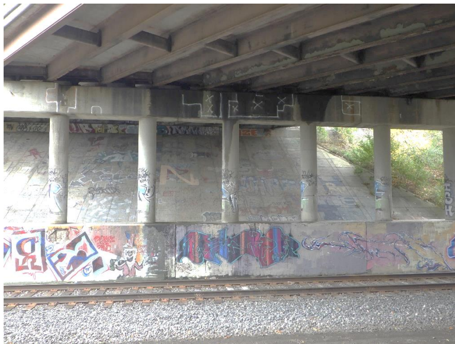
Photograph No. 24 North Side of South Pier (Pier 1), Center Portion
