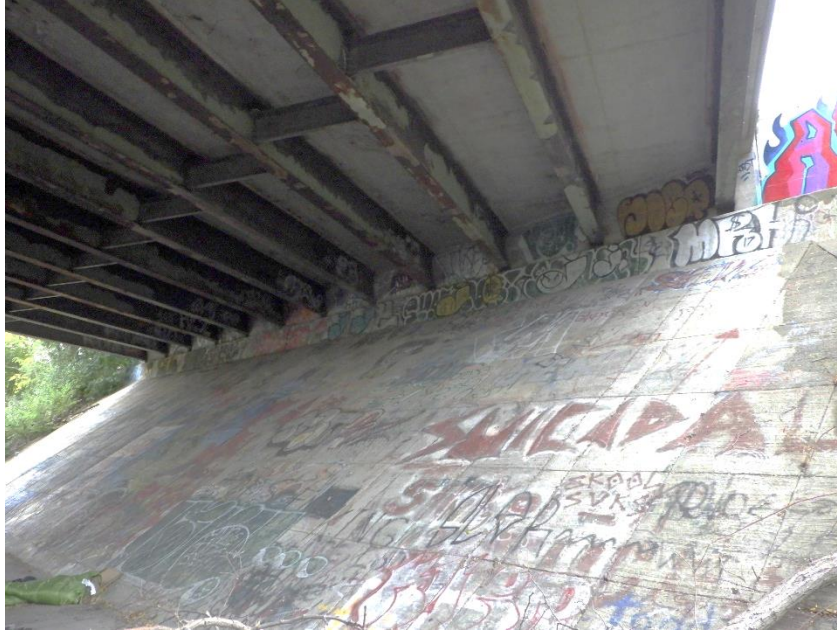
Photograph No. 17 North Abutment and Slope Paving
