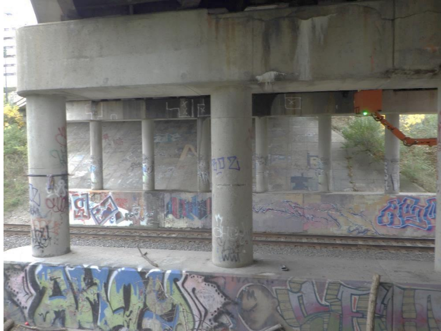
Photograph No. 21 West Portion of North Side of North Pier (Pier 2)
