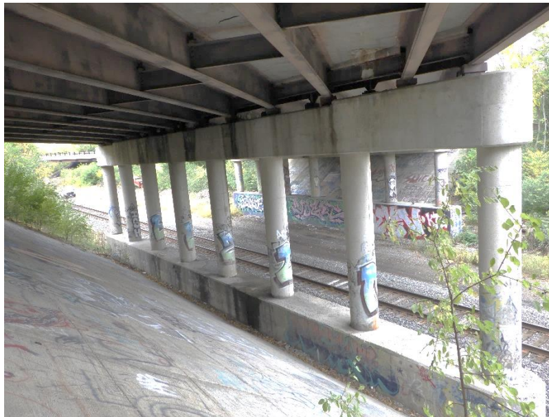
Photograph No. 22 South Side of South Pier (Pier 1)
