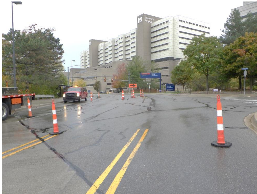
Photograph No. 2 South Approach Looking South
