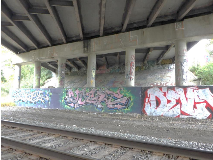
Photograph No. 19 South Side of North Pier (Pier 2)
