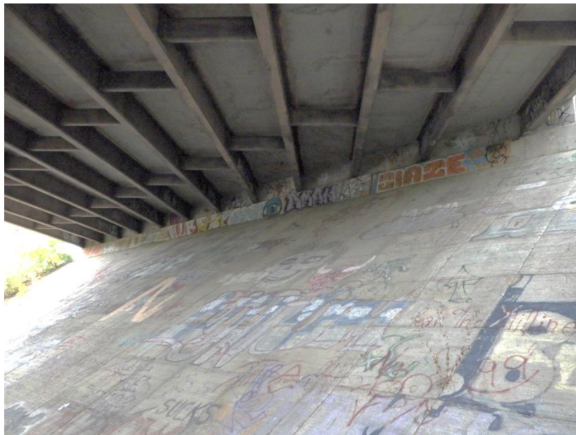
Photograph No. 18 South Abutment and Slope Paving
