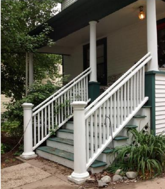
Figure 1. Porch Stair & Rail Overview
