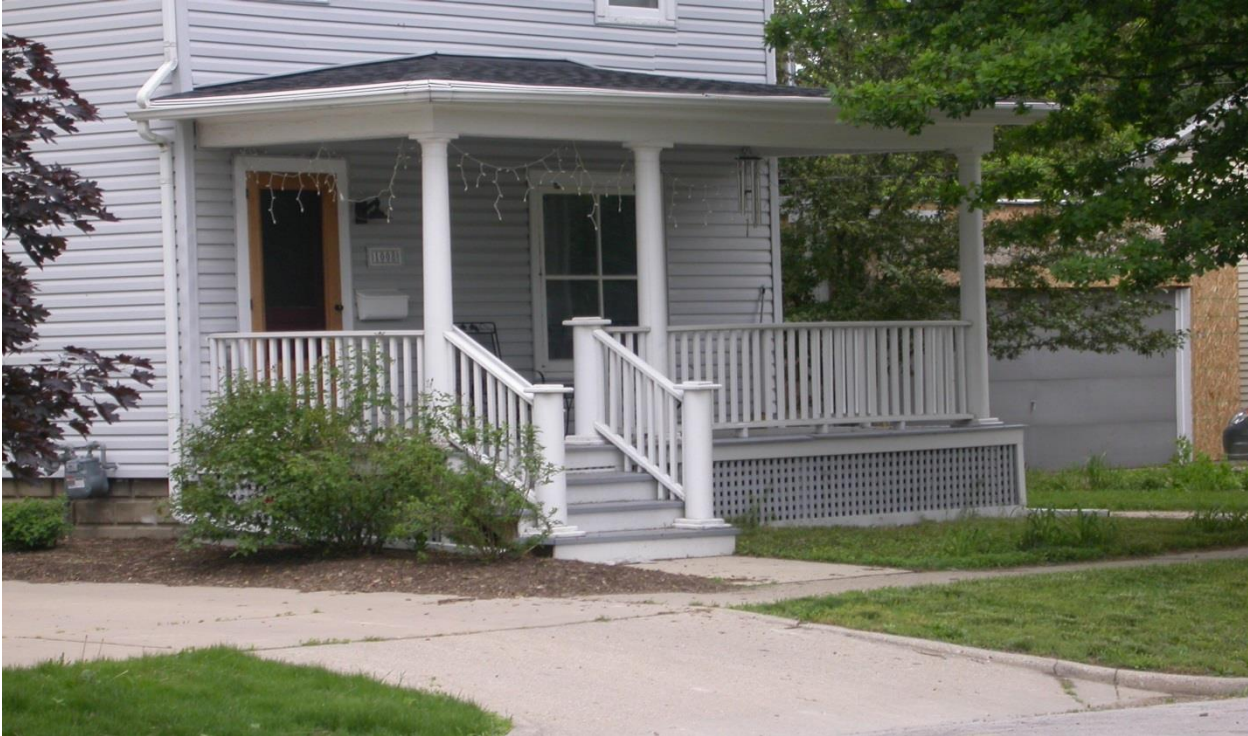
Figure 7. Washington Street Representative Style of Porch Skirting & Graspable Handrail
