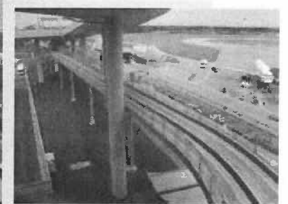
Lightweight pods allow the guideway support structures (shown above) to be much smaller than those constructed for typical roadways, which can reduce the visual impact
