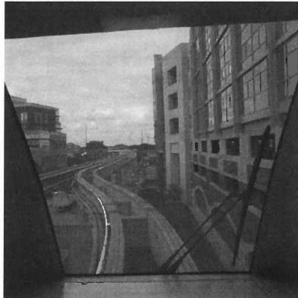
The Clarian People Mover uses two separate parallel elevated guideways, both of which operate in both directions
