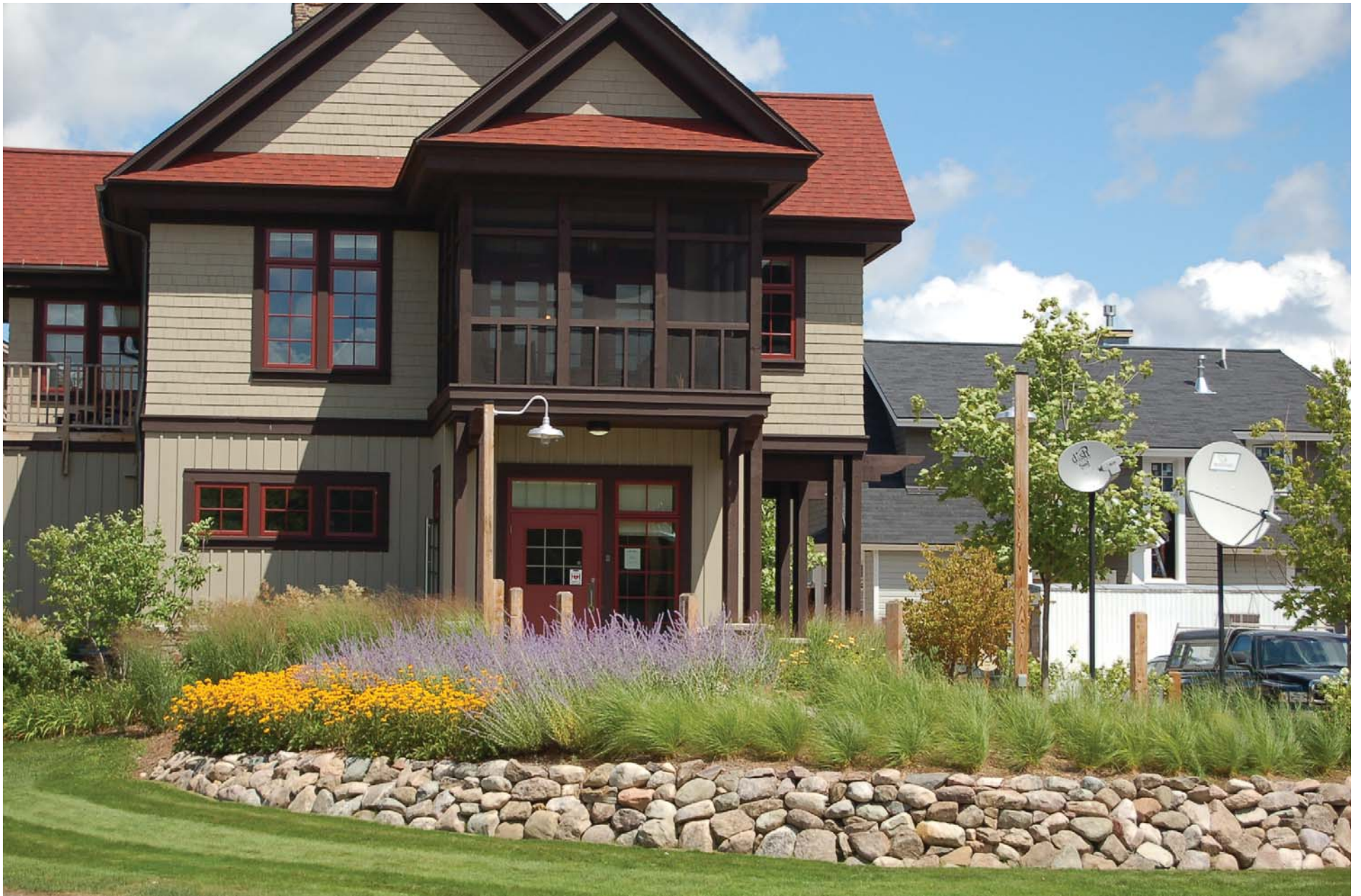
Dry laid stone/rock retaining wall: Low stone retaining walls at street will be similar to the one pictured above.
