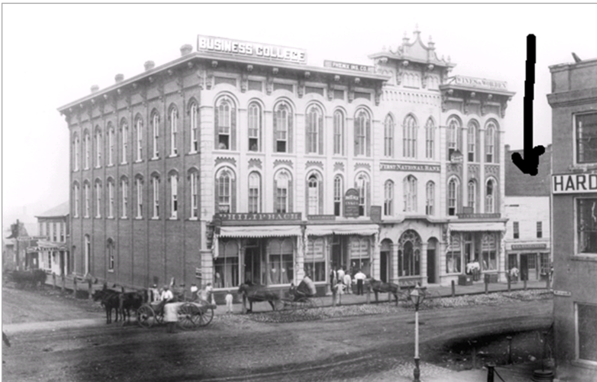
1867 Photo of 120-126 South Main (arrow points to future location of 118 S Main)
