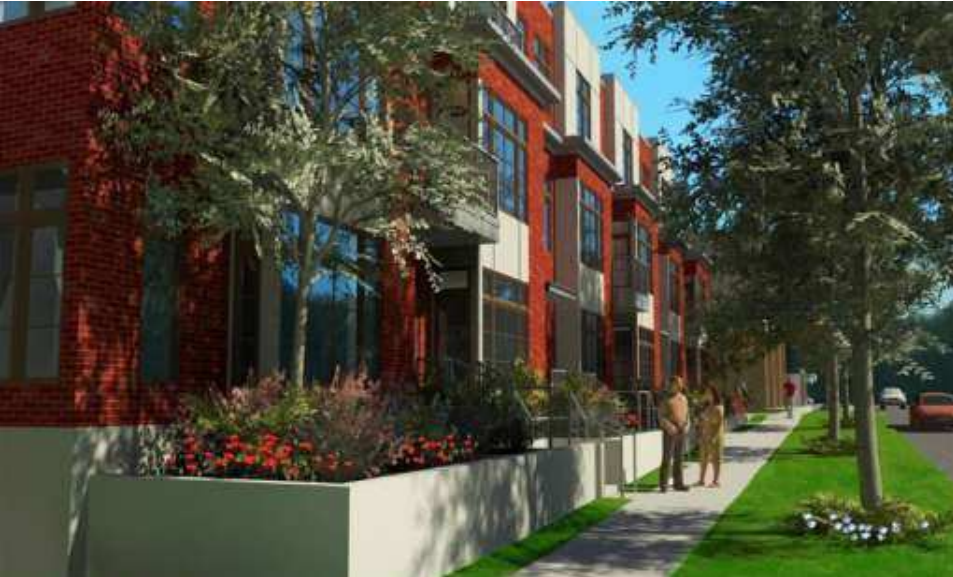
414 North Main under construction
