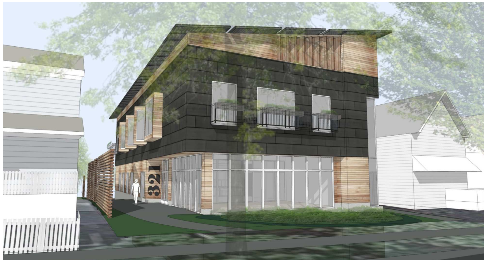
View from the southeast
