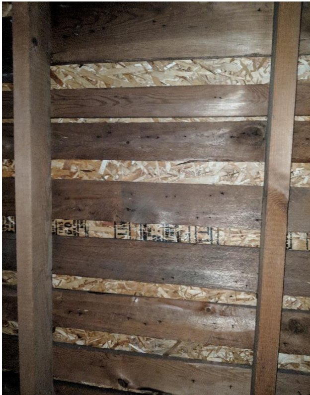
Roof Framing: Attic, rafters are 2" x 4"@ 24" OC
