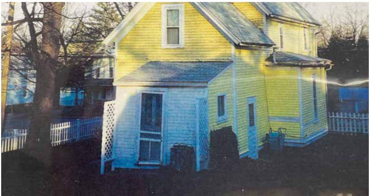
ORIGINAL WEST VIEW
