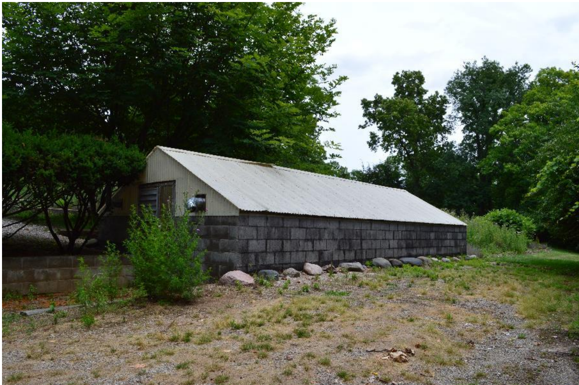
10 - Looking northeast at coldhouse, July 2017
