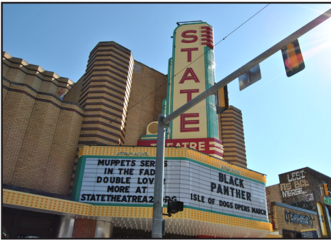
Name: State Theater Renovation Occupancy: A-1 Assembly Theater Location: Ann Arbor, MI
