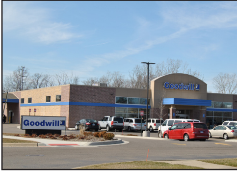
Name: Goodwill Store Occupancy: M-Mercantile Location: Pittsfield Township
