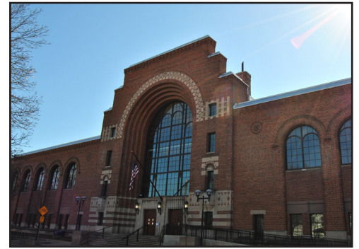
Name: IM Building Renovation Occupancy: A-2 Recreational Location: U of M Campus Ann Arbor
