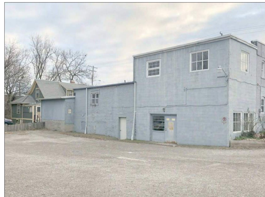
VIEW OF EXISTING WEST ELEVATION FROM THE SOUTH WEST - 2
