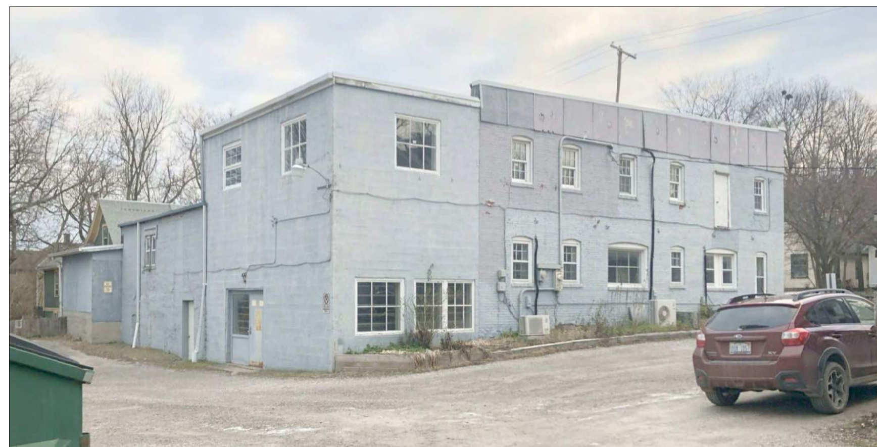
VIEW OF WEST & SOUTH ELEVATIONS FROM THE SOUTHWEST - 1
