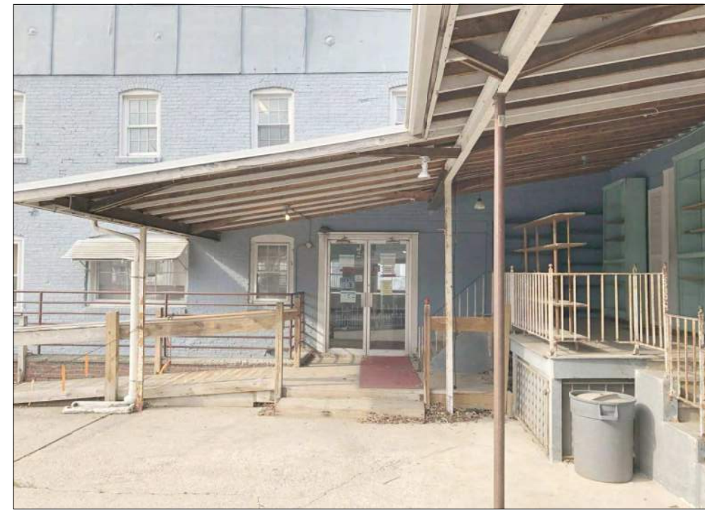
VIEW OF EXISTING NORTH ELEVATION, UNDER SHED ADDITION
