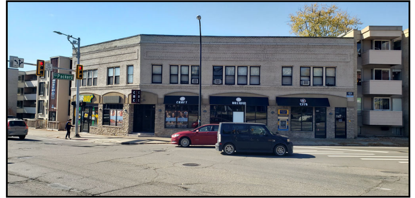
VIEW OF BUILDING AT NW CORNER OF S. STATE & PACKARD STREETS
