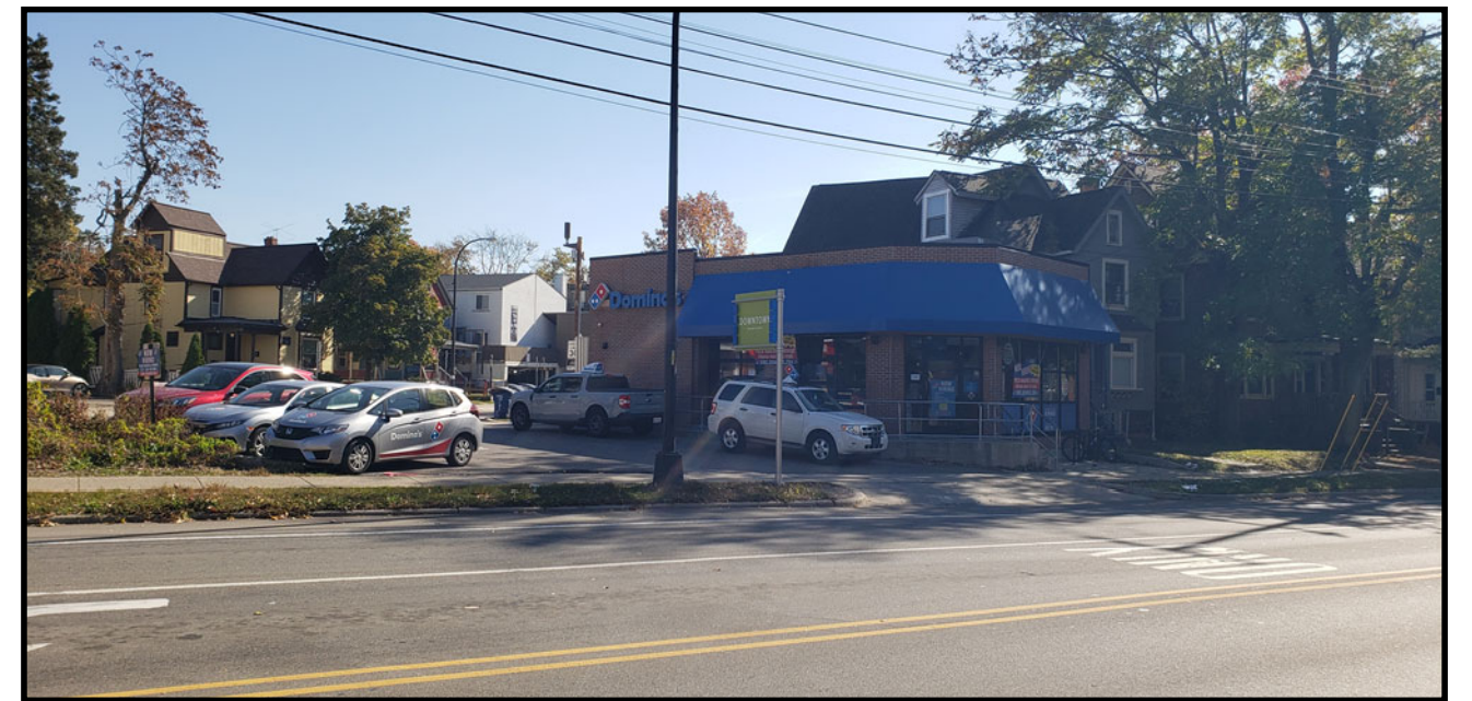
VIEW LOOKING SW AT INTERSECTION OF S. STATE & PACKARD STREETS
