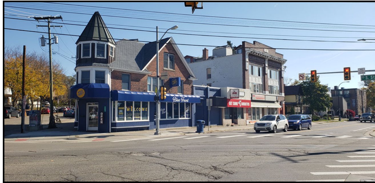
VIEW LOOKING SOUTHWEST FROM SE CORNER
