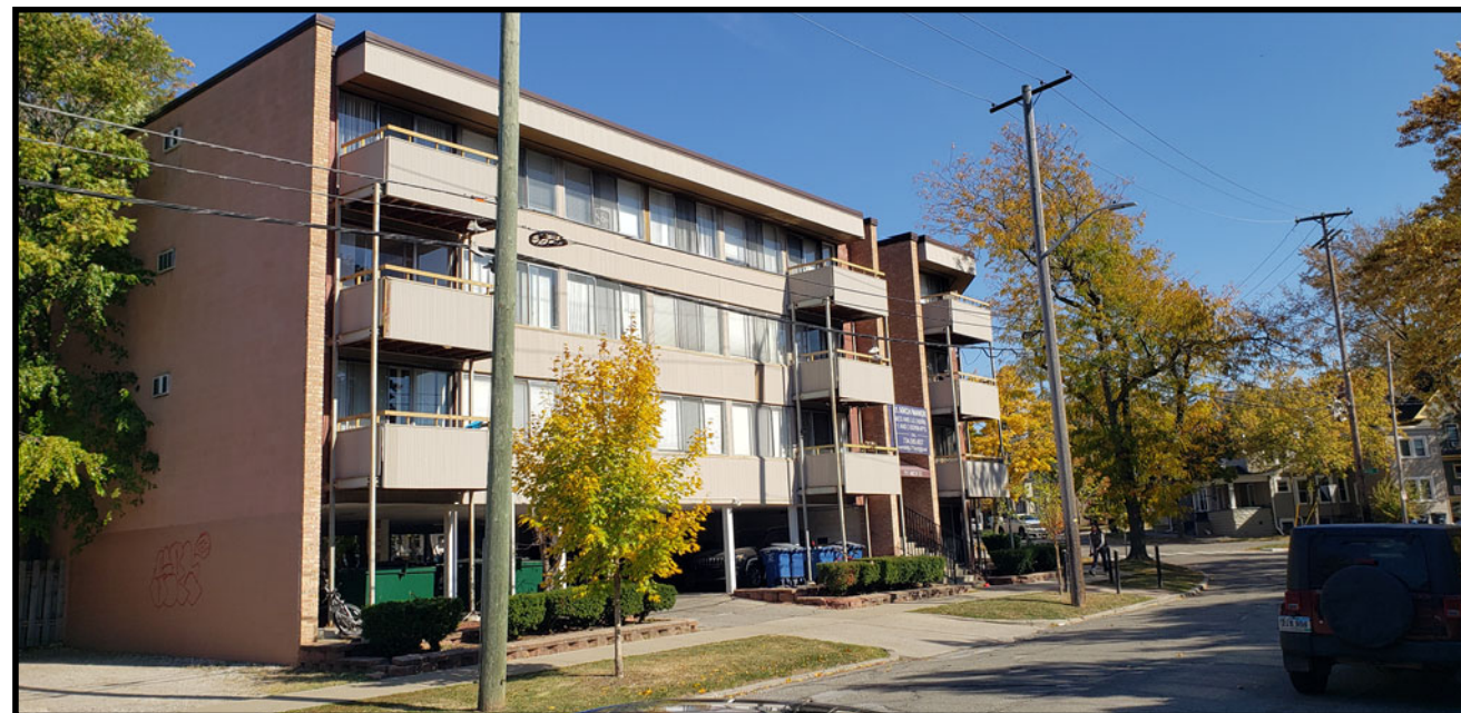
VIEW FROM ARCH STREET LOOKING NORTHEAST
