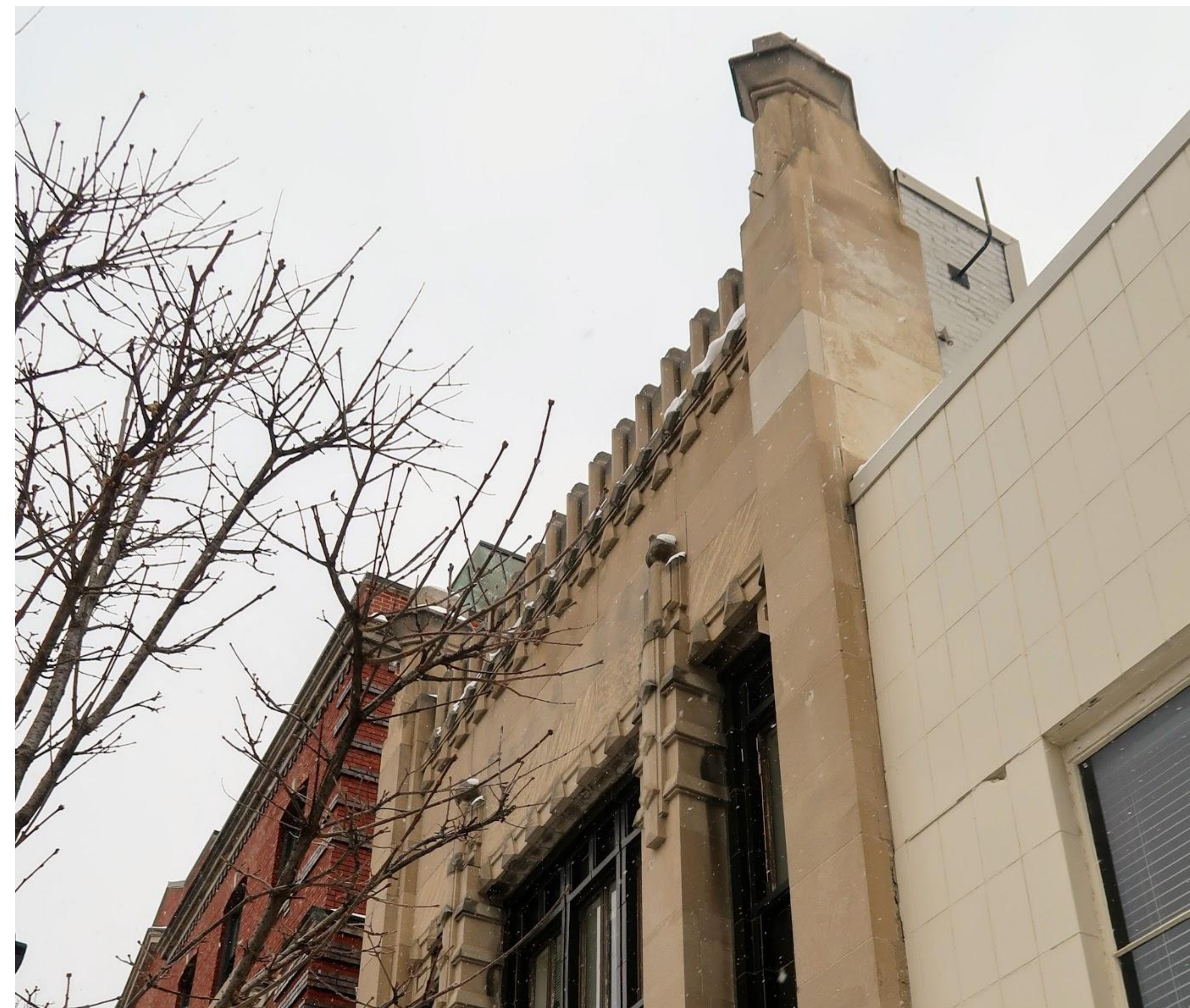
Facade Detail from adjacent sidewalk
