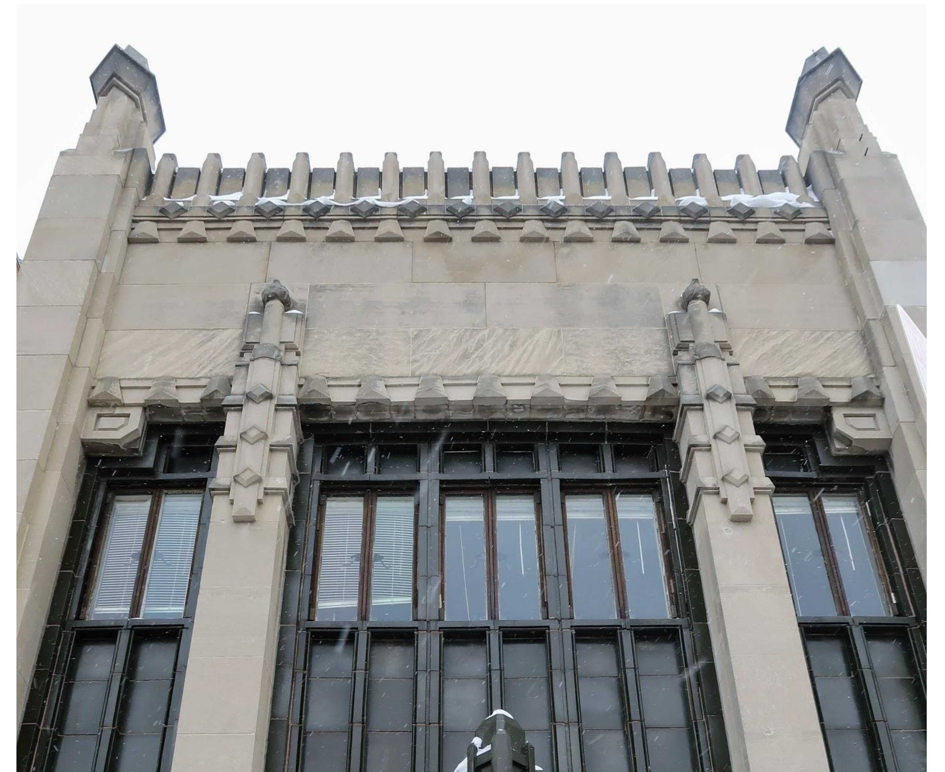
Facade Detail from adjacent sidewalk
