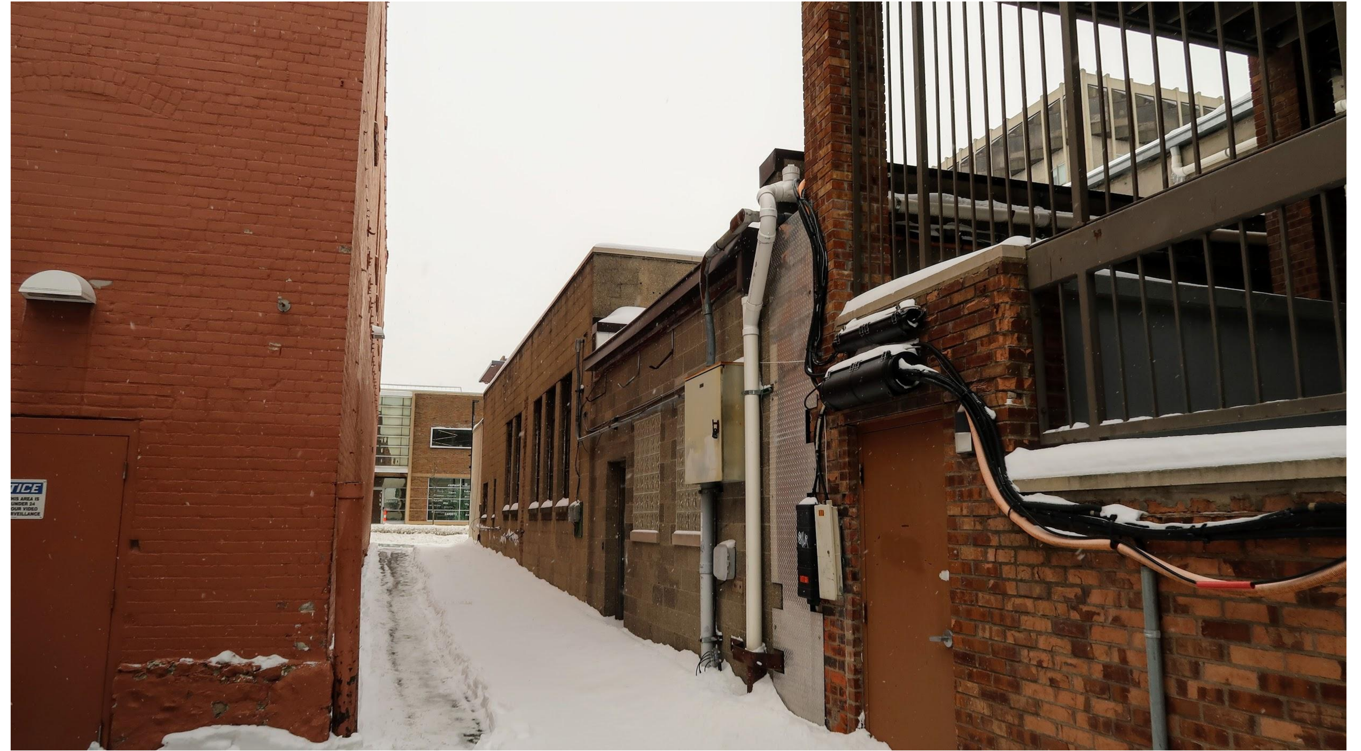
Back side of building (1949 Addition) from south-facing alley.
