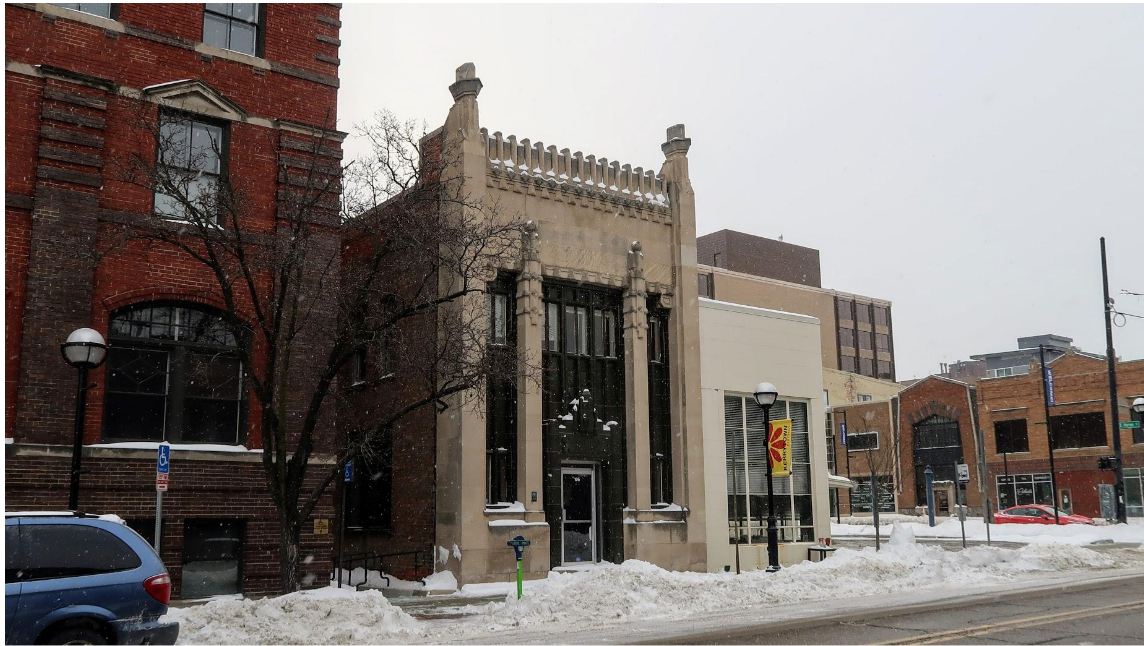
Facade from across N. 4th Ave, showing ally.
