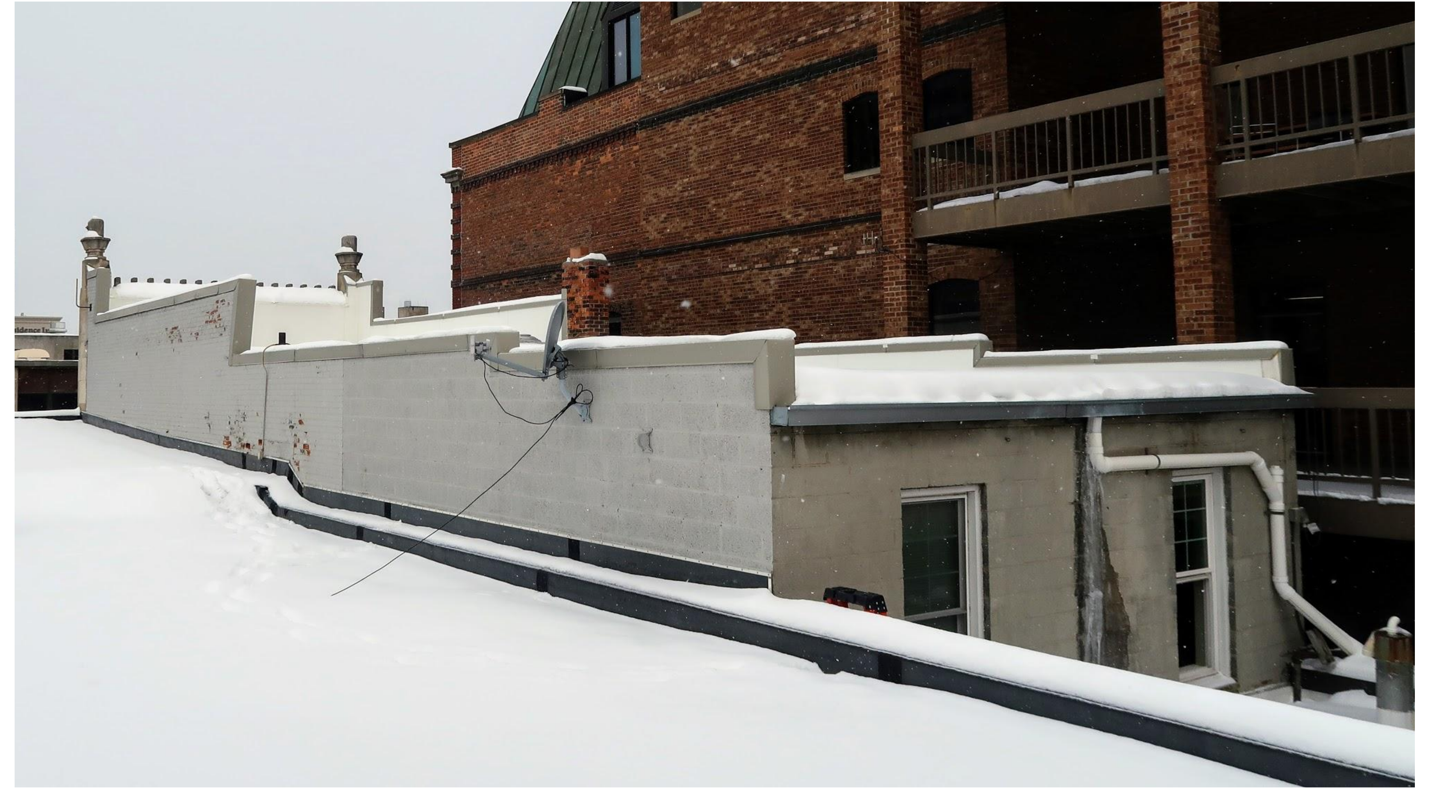
Backside roof including 1949 addition.
