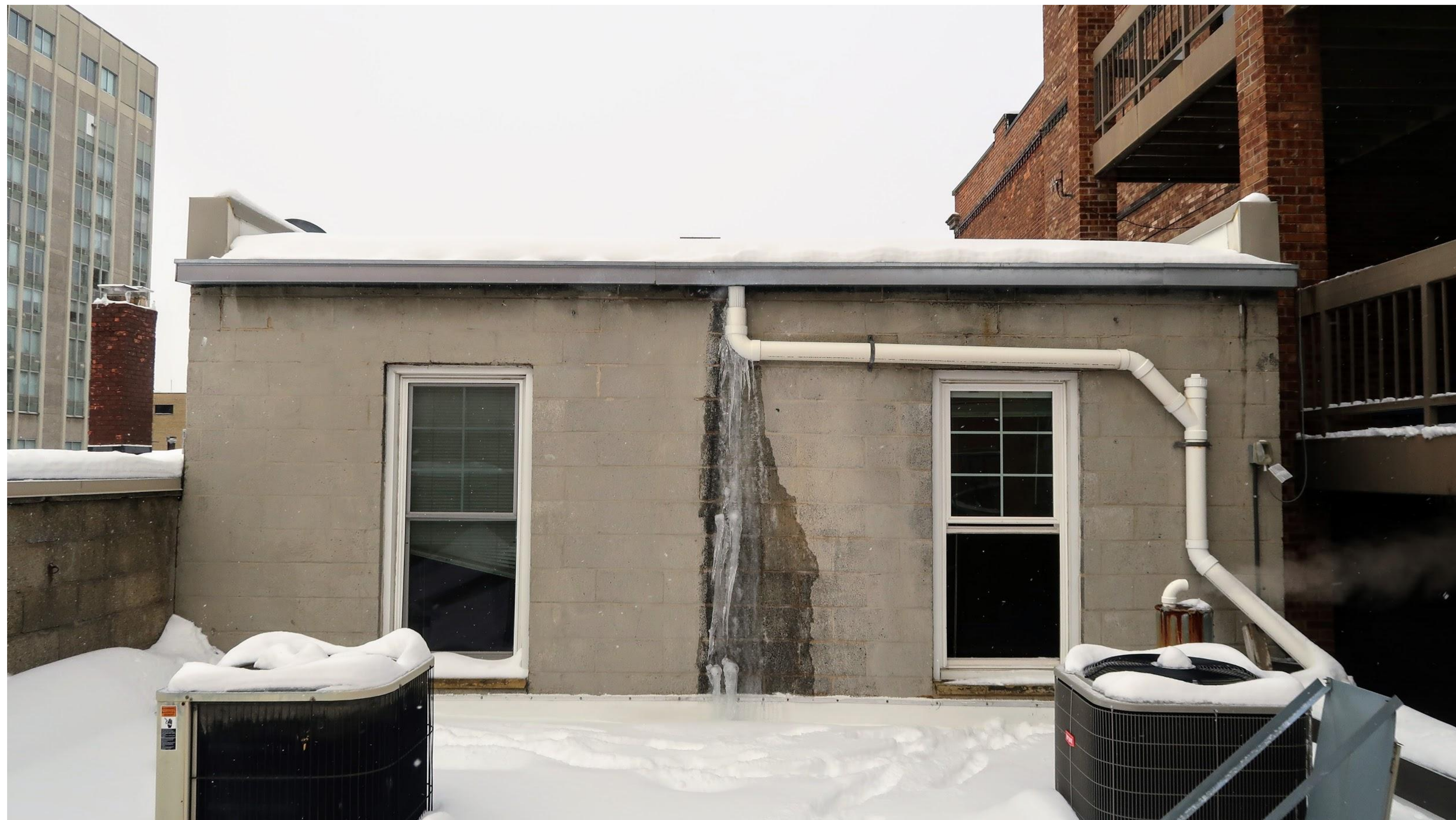
Backside roof including 1949 addition.
