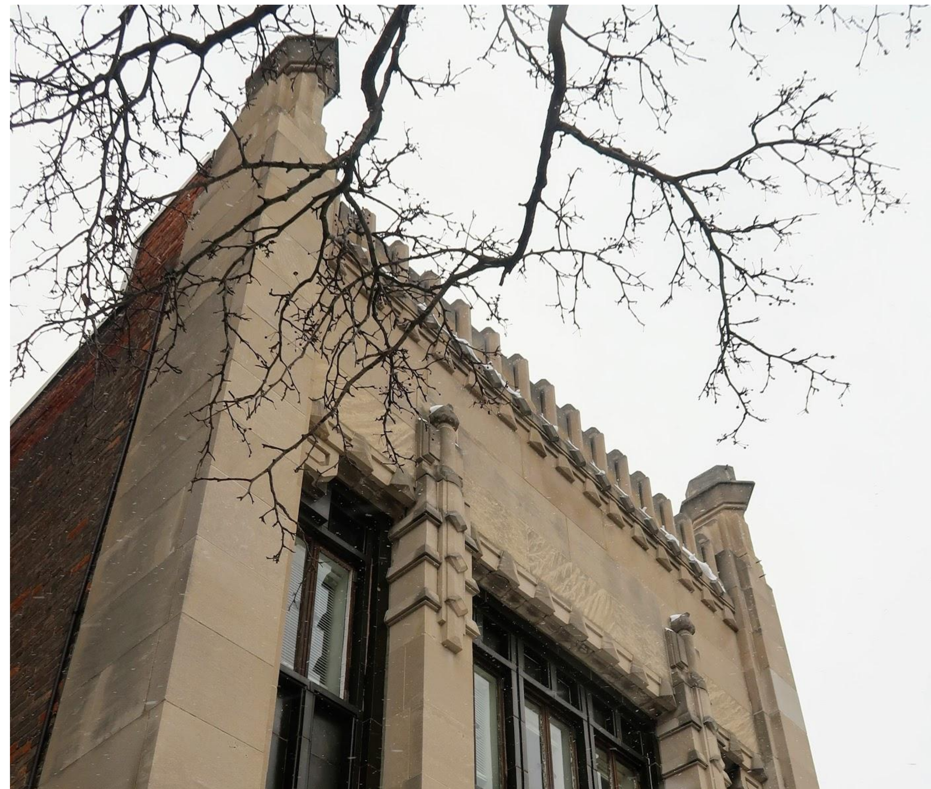
Facade Detail from adjacent sidewalk
