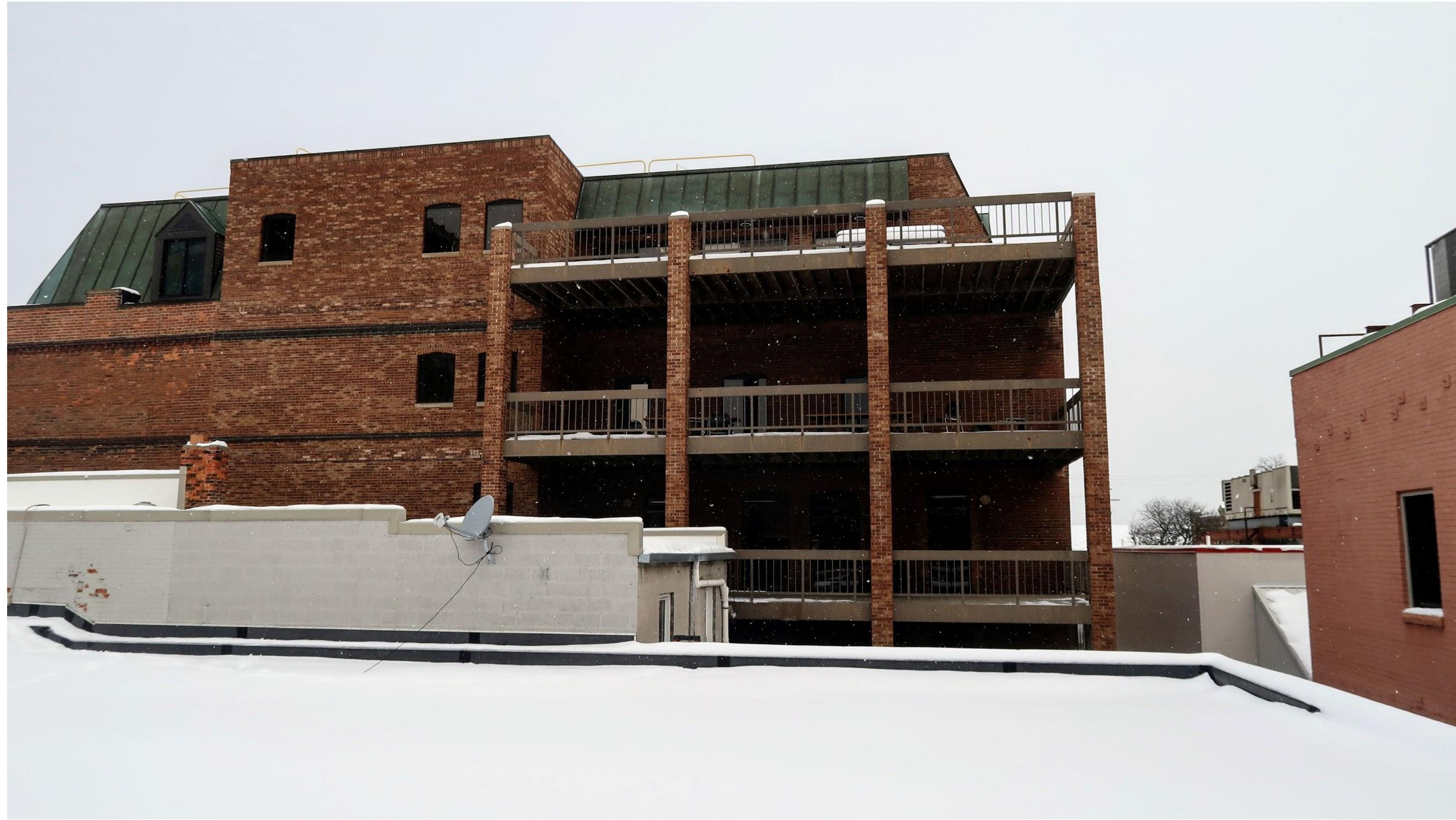
Backside roof and parapet including 1949 addition.
