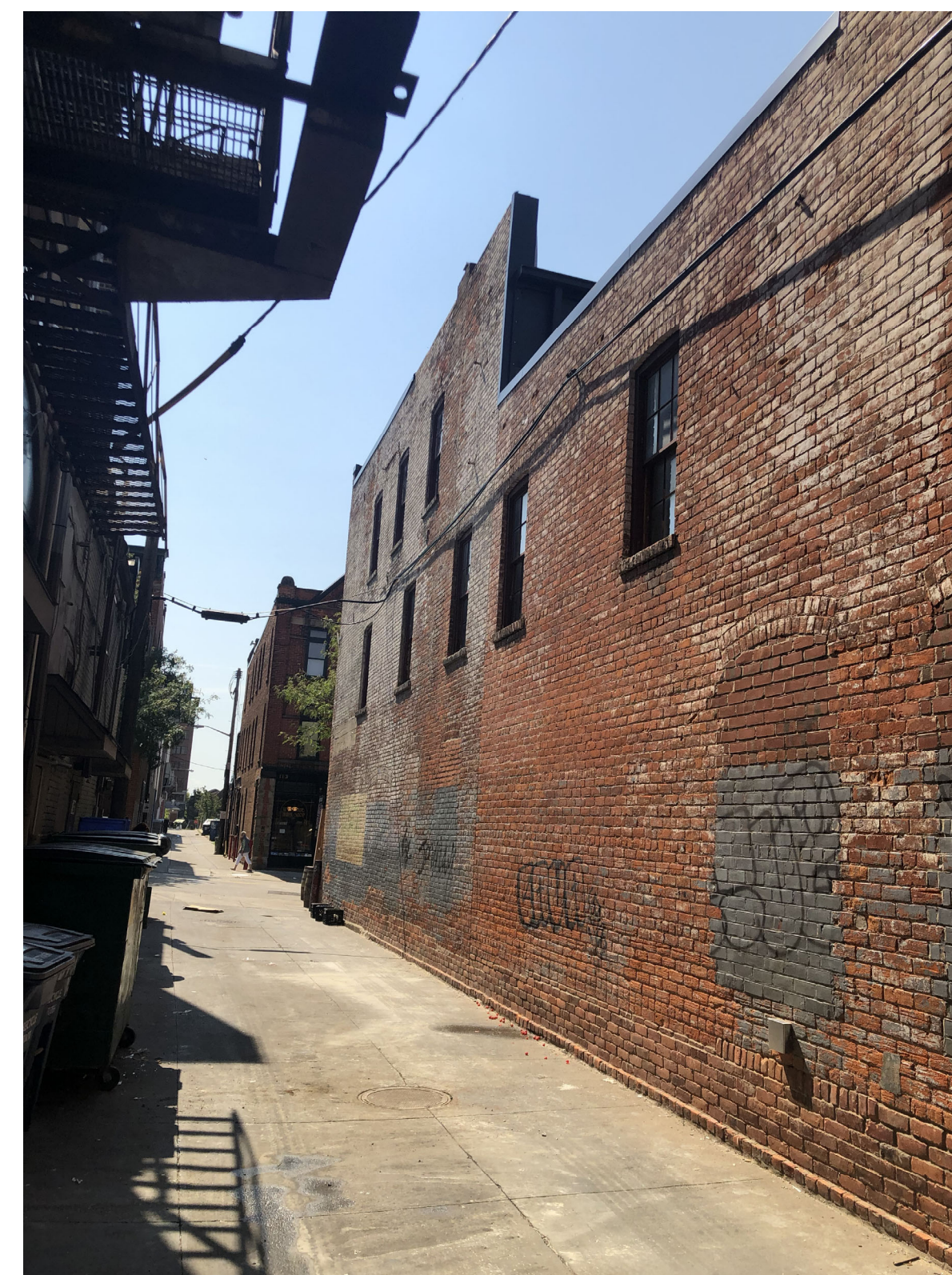
2 SITE PHOTO LOOKING SOUTHWEST N.T.S.
