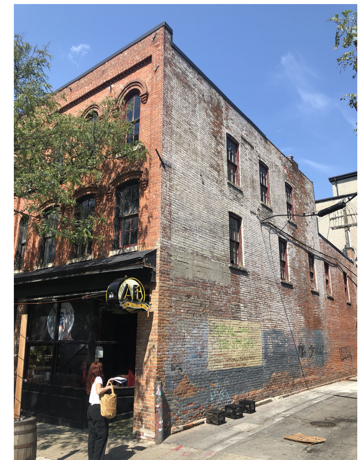
1 SITE PHOTO LOOKING NORTHWEST N.T.S.
