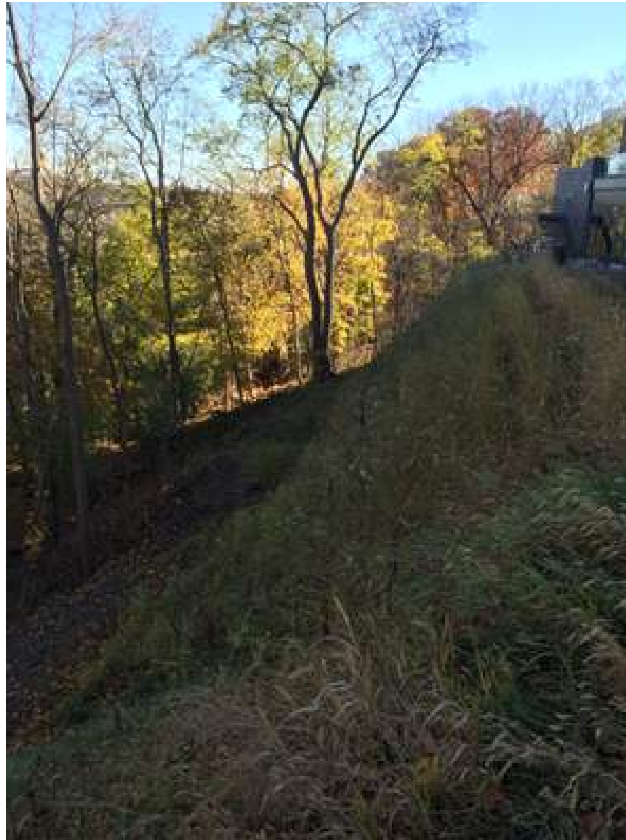
EXAMPLE: MSE WALL AFTER ESTABLISHING VEGETATIVE GROWTH PHOTO COURTESY SME - UNIVERSITY OF MICHIGAN SCHOOL OF NURSING
