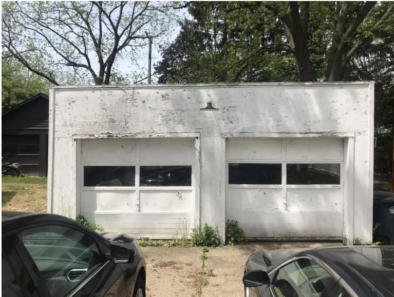
Photo of East Elevation
