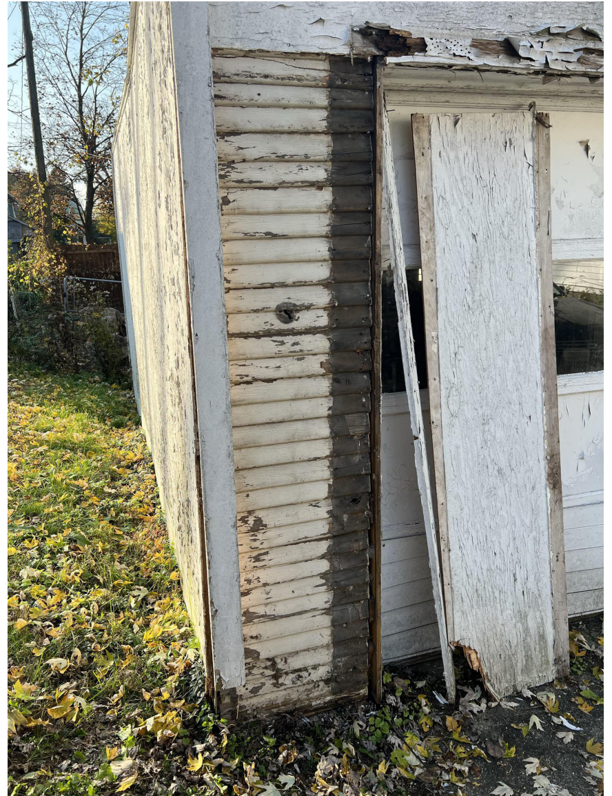
Photo of removed plywood covering with historic cladding exposed.
