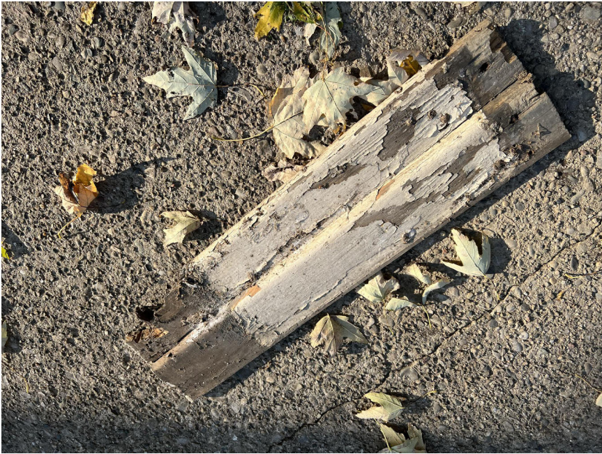
Photo of front of historic cladding from garage.
