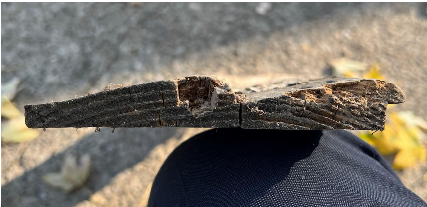
Photo of profile of historic cladding from garage.
