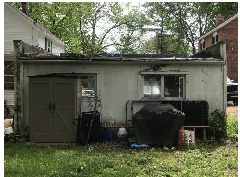
Photo of West Elevation
