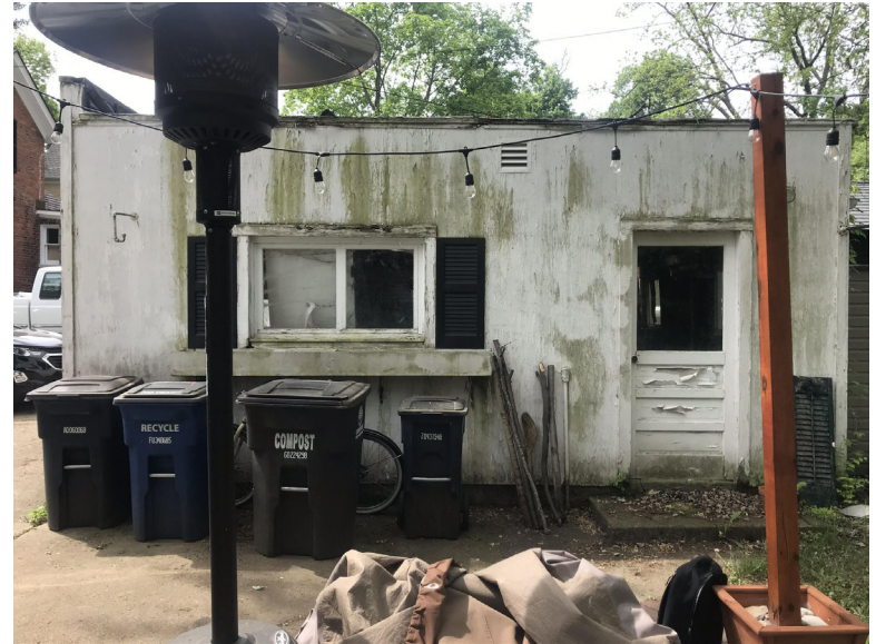
Photo of North Elevation
