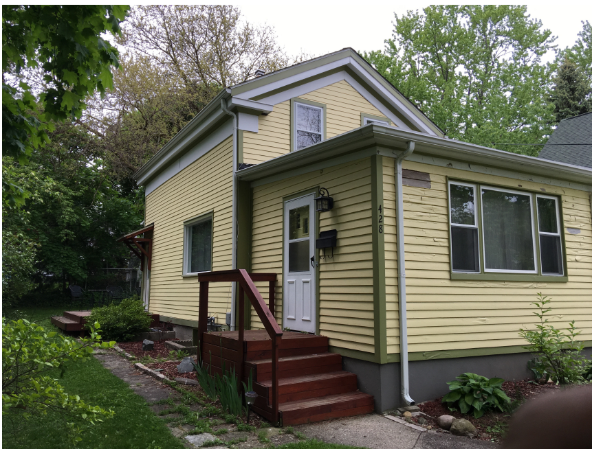
South Elevation – Existing Entry Door
