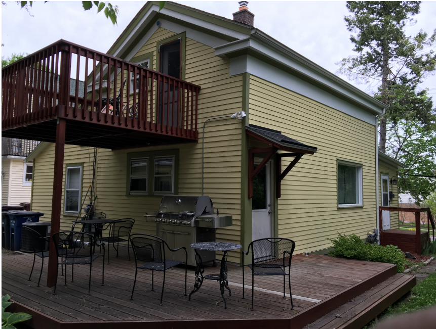
West Elevation - Windows and Deck
