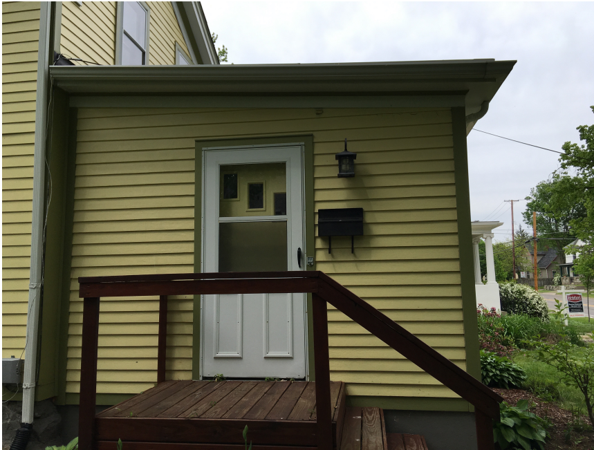
South Elevation – Existing Entry Door
