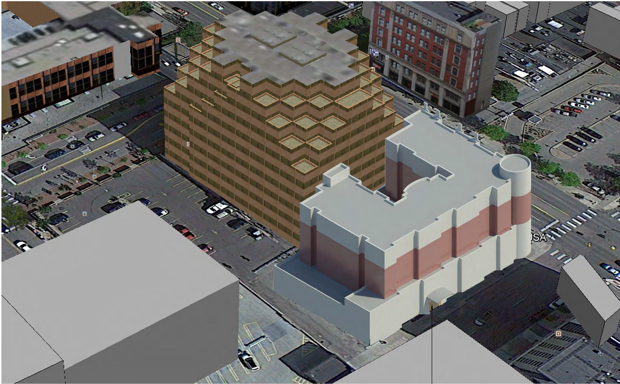
ARIAL VIEW FROM NORTH
