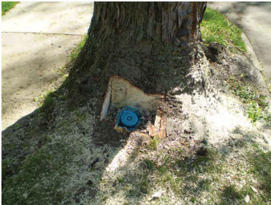
The base of this street tree had to be cut to access the water curb stop box to repair a resident’s water service. To avoid future conflicts, Forestry staff and city tree planting contractors now coordinate with Miss Dig and City utility staff to locate all underground utilities prior to planting. New trees are planted at least 8 feet from underground utility service lines and access points.
