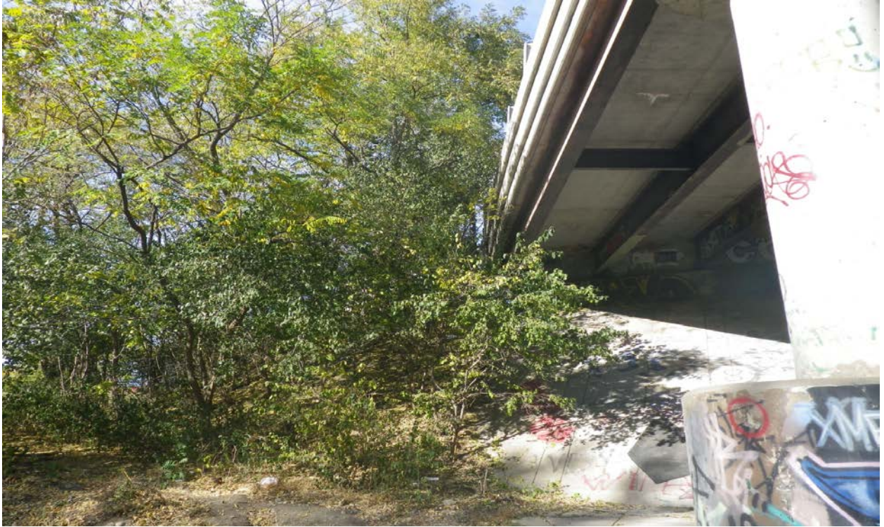
Figure 15 Typical heavy vegetation surrounding bridge
