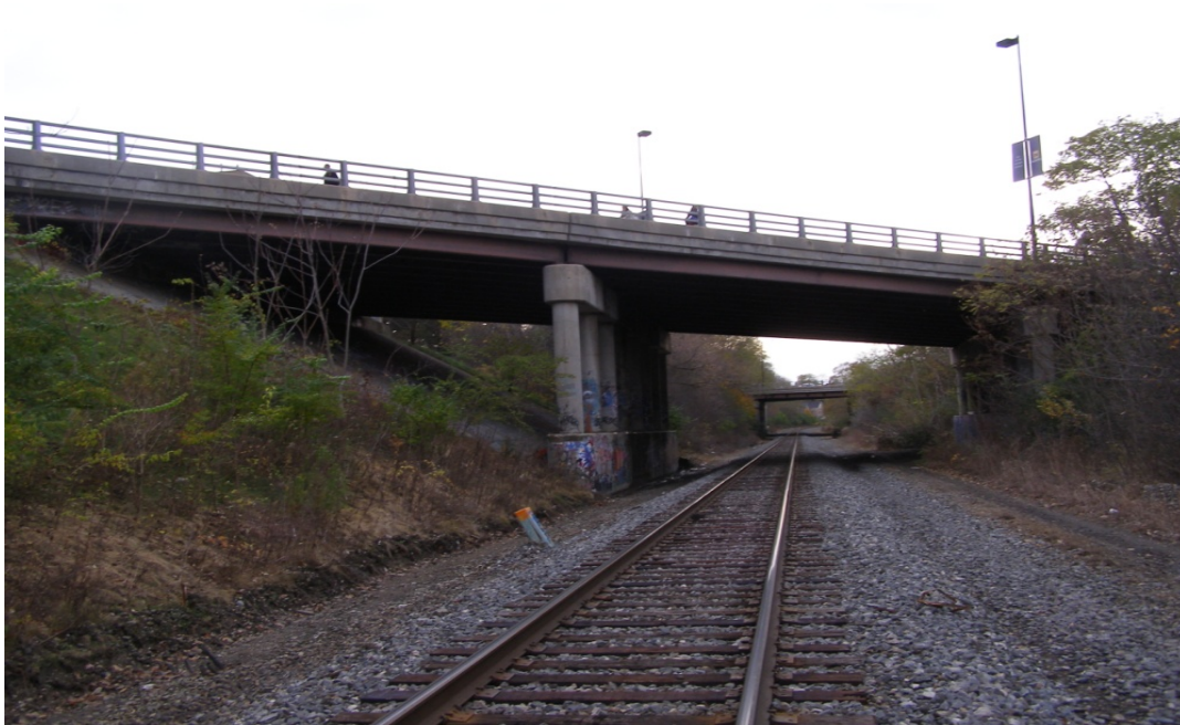
Figure 1 East Elevation Looking West
