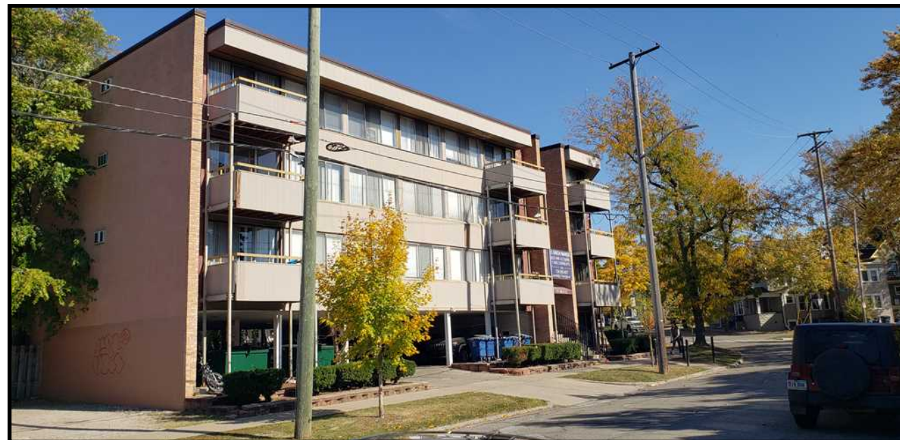
VIEW FROM ARCH STREET LOOKING NORTHEAST
