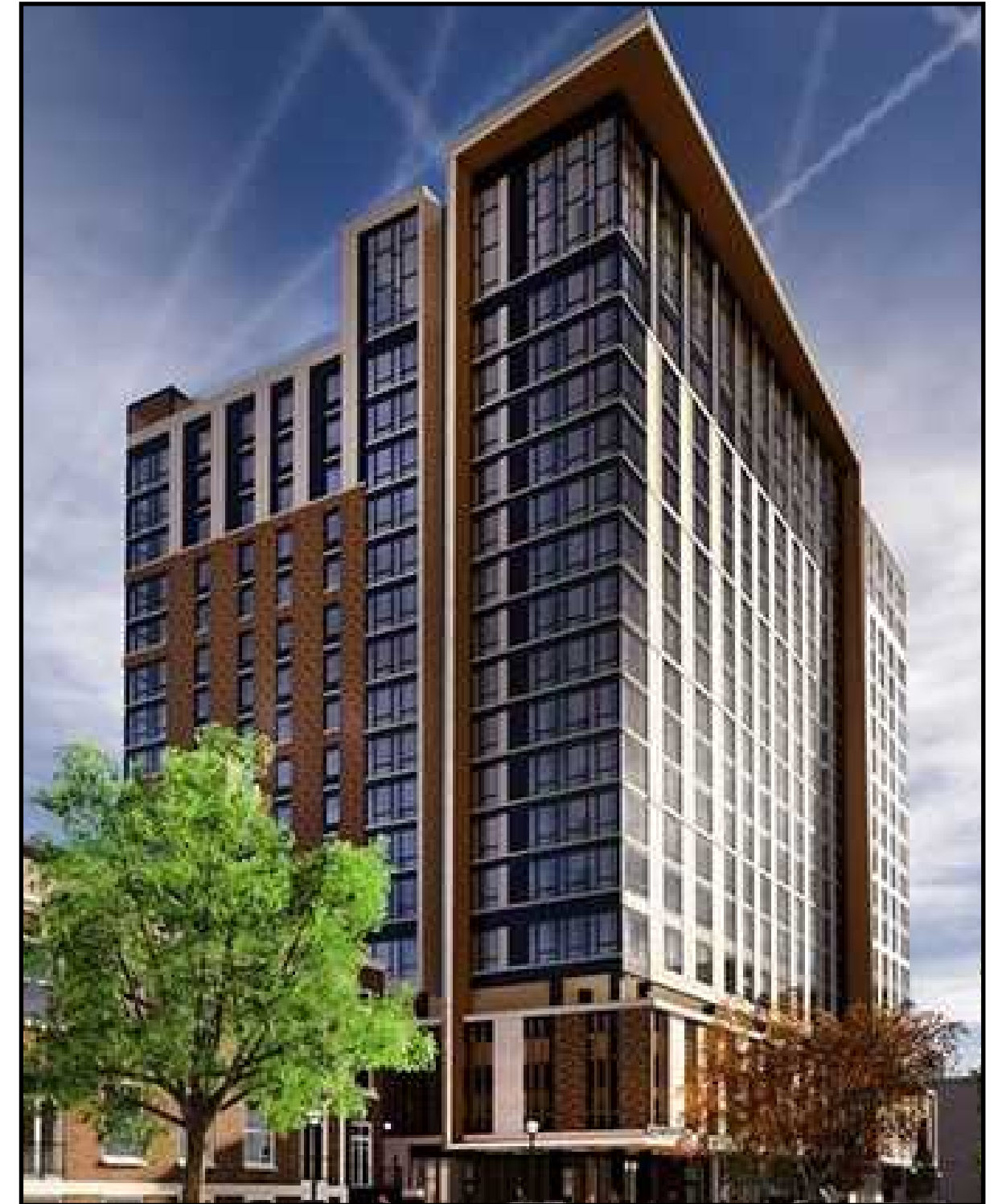
616 EAST WASHINGTON STREET (19 STORIES) 616 EAST WASHINGTON STREET
