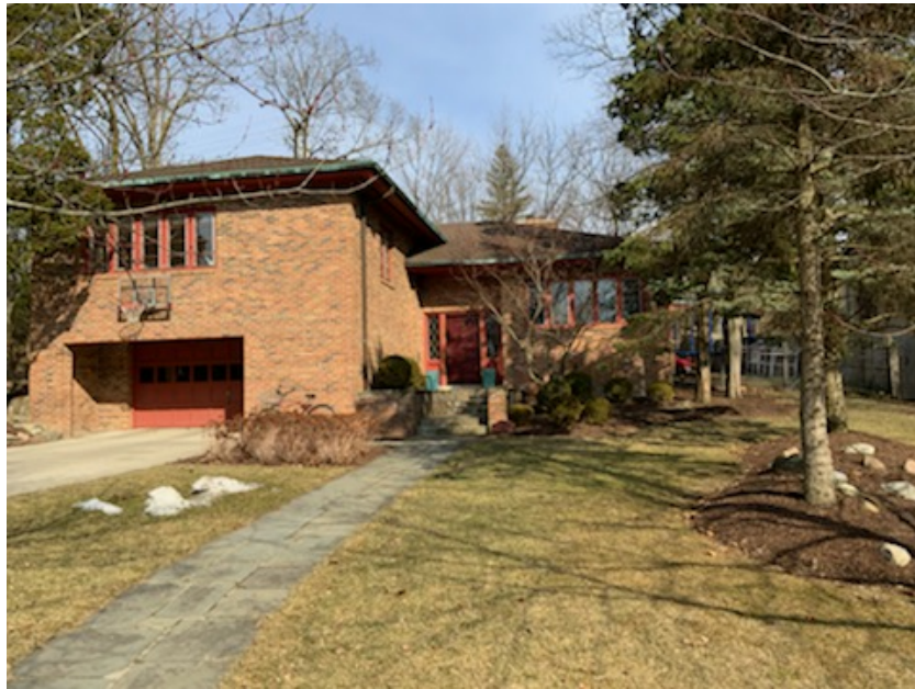
Existing west elevation and entry
