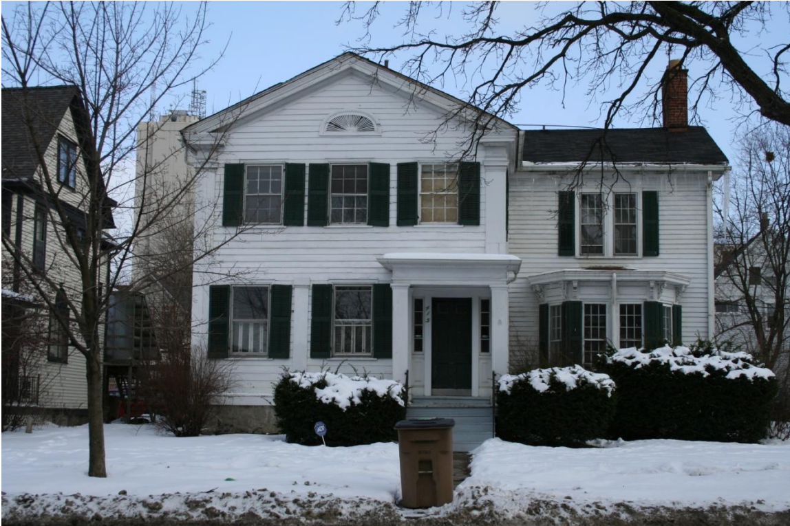
Photograph 6 – 415 South Fifth Avenue, Gaskell/Beakes House, February, 2010
