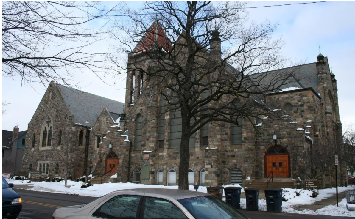
Photograph 4 – 423 South Fourth Avenue, Bethlehem Evangelical Church, February, 2010
