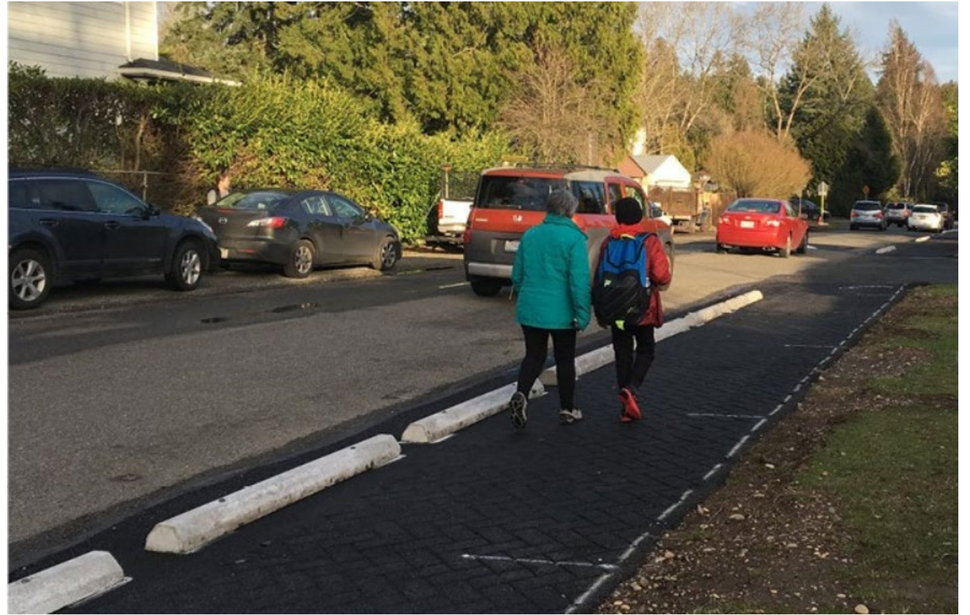
At-grade interim asphalt walkway (Source: Seattle Department of Transportation)
