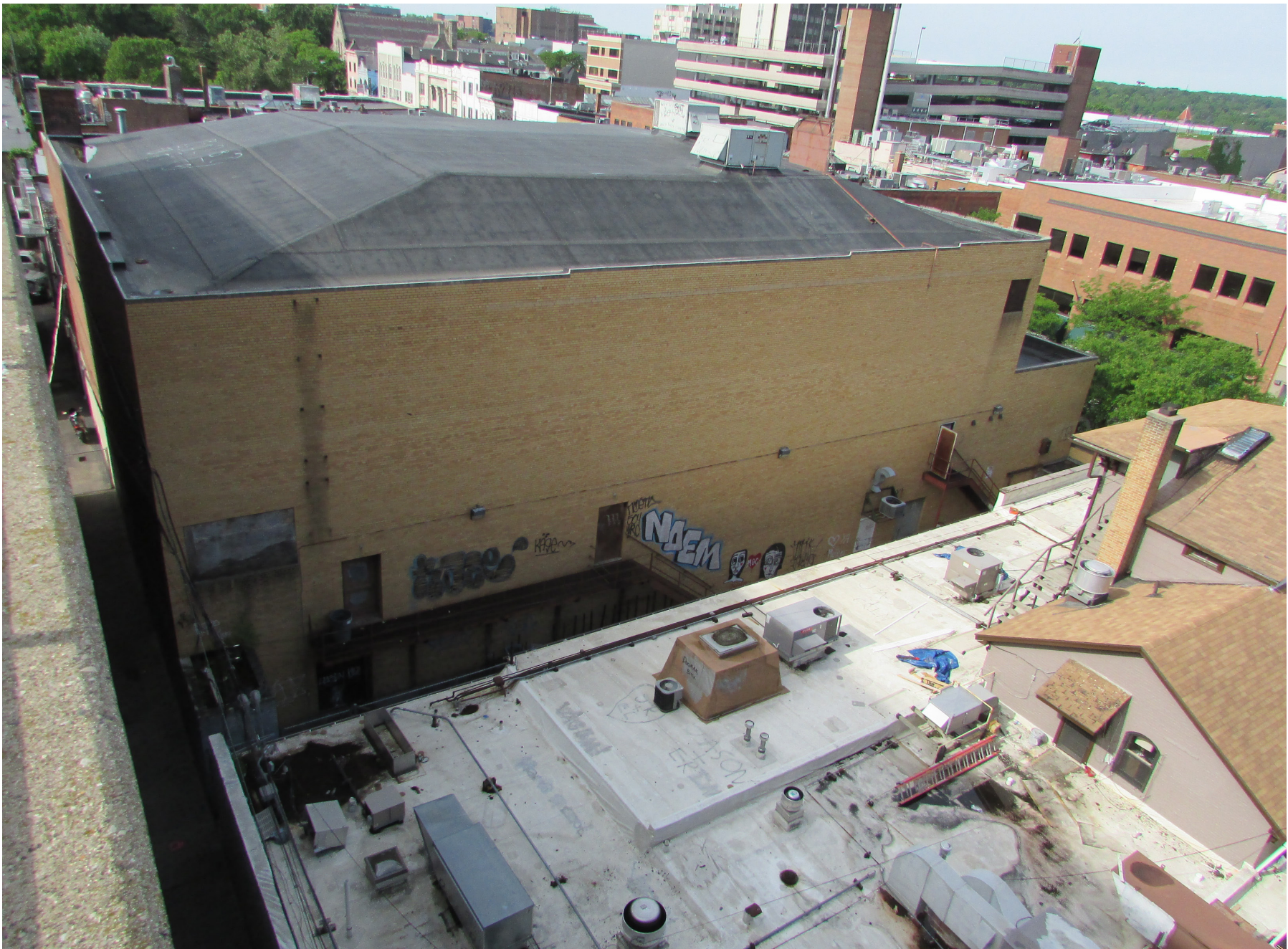
current view of North alley/ facade - 2016
