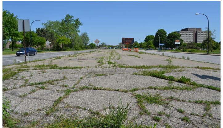
Concrete medians dominate the landscape in Area 2
