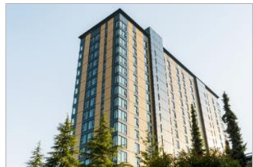
Figure 28. Brock Commons Tall Wood The first mass hybrid timber residential high-rise building in North America.
