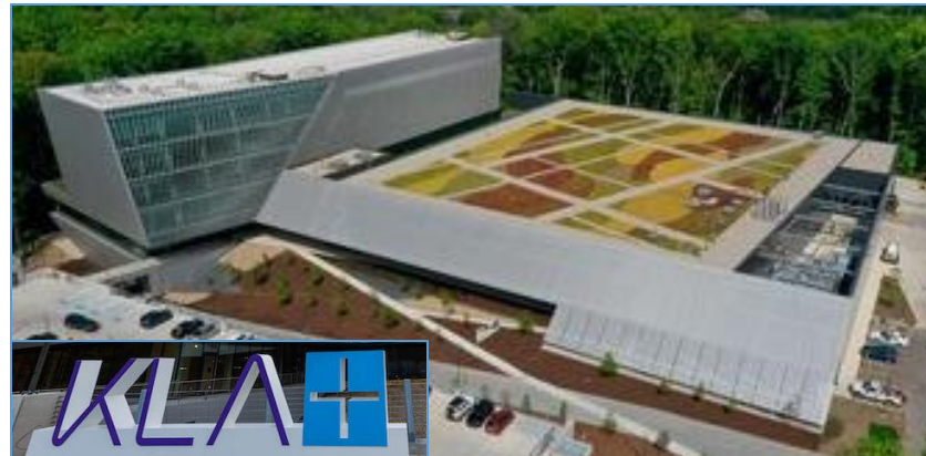
Figure 11. Semiconductor Company KLA's Ann Arbor, Michigan Campus, $200M Second US Headquarters, Cleanroom and R&D Center
