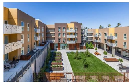
Figure 27. Mayfield Place, Palo Alto, CA
