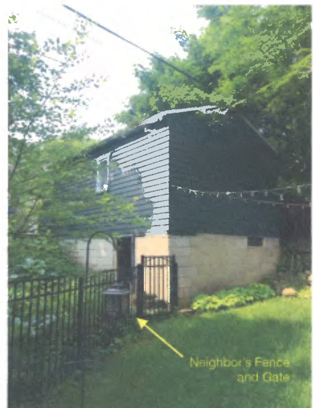
NorthEast View (View From 315 W. Davis)
