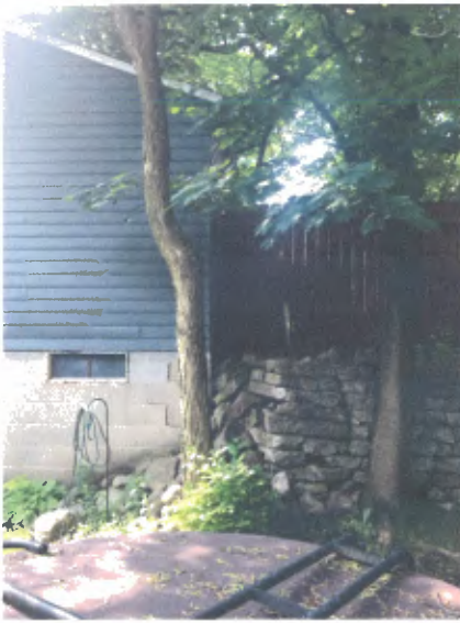
Close-Up of Neighbor's retaining wall abutting up to garage
