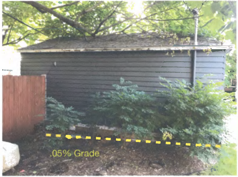
West (Side) Elevation View from 302 W. Hoover
