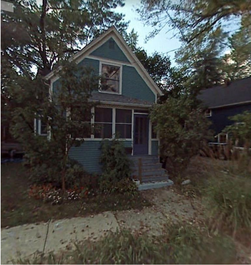
224 Murray Avenue (November 2020, Google Street View)
