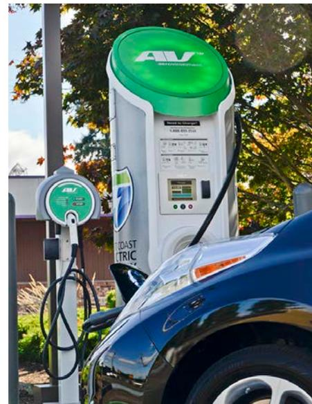
Photo 13. One of many side by side DCFC and Level 2 EVSE installed along the West Coast Electric Highway in Oregon and Washington. *Photo from Washington State Department of Transportation (WSDOT).*
