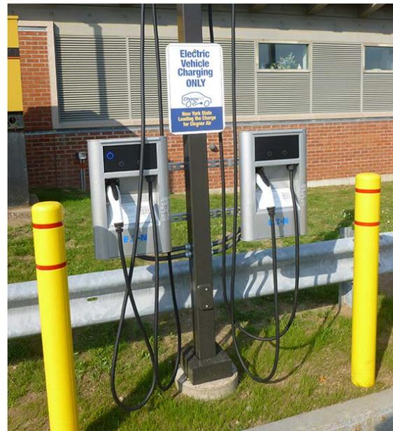
Photo 17. These two EVSE are located close to the building, reducing trenching costs. *Photo from NYSERDA.*
