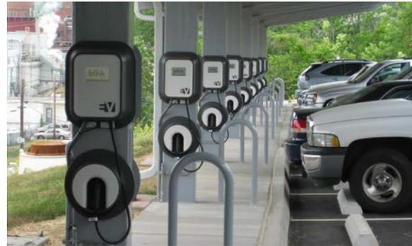
Photo 1. This series of Level 2 EVSE were installed by the EV Project. *Photo from INL.*
