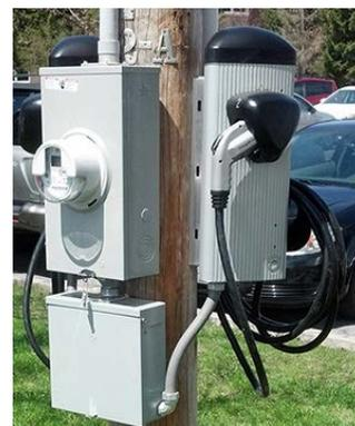
Photo 20. An electrical meter mounted alongside the EVSE and connected with conduit.
