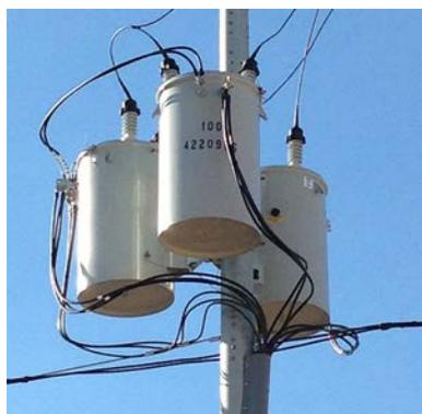
Photo 22. Step-down transformer located at the utility service point.
