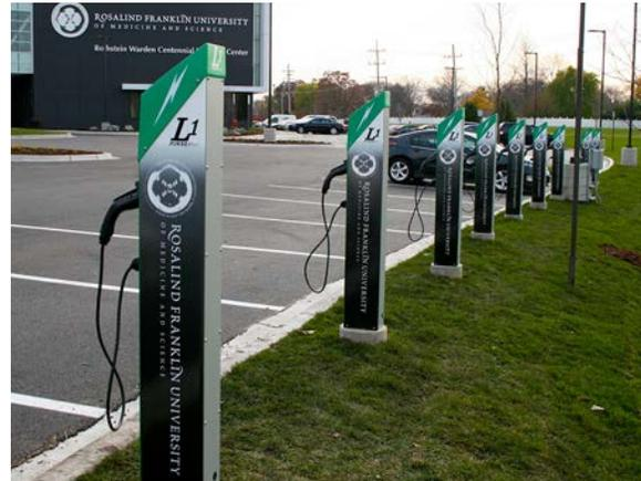
Photo 12. Level 1 pedestal EVSE at Rosalind Franklin University in Illinois. *Photo from Telefonix.*
