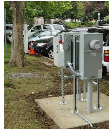
Photo 9. Electrical meter and switch servicing Level 2 EVSE.
