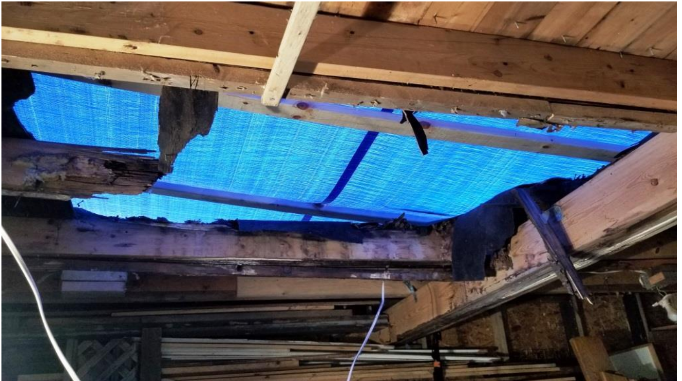
RECENT ROOF DAMAGE DUE TO ROT AT SHALLOW SLOPED ROOF
