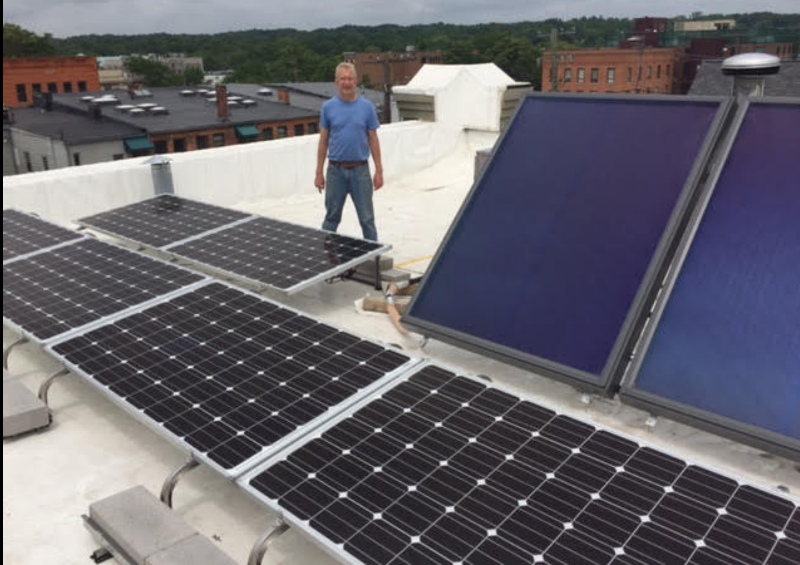
PV panels and hot water panels on our white roof, in downtown Ann Arbor.
