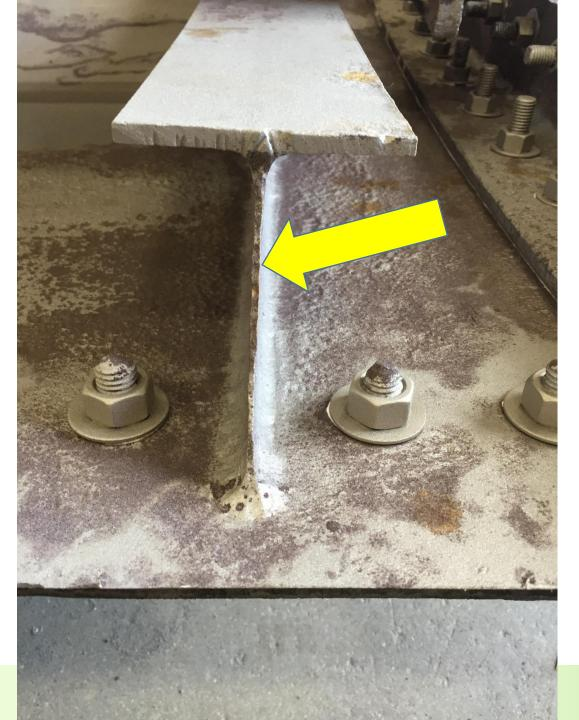
• Significant section loss in structural steel members due to corrosion
