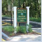
A physical landmark that indicates a change from a higher speed arterial road to a lower speed residential or commercial district.
