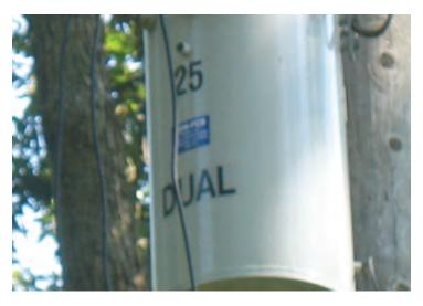
Viewing the non-PCB containing label located on the previously mentioned pole-mounted transformer.
