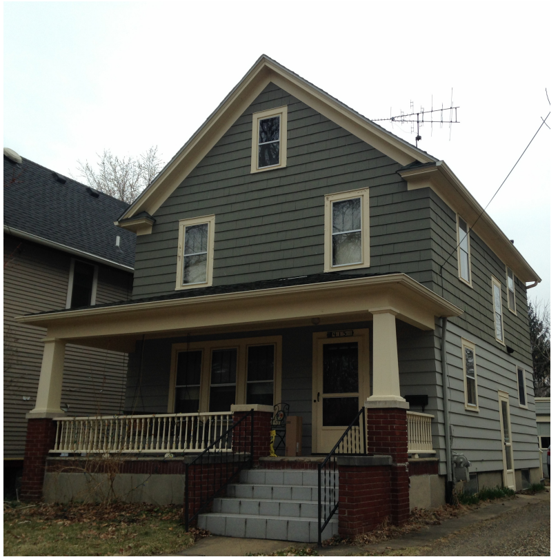
VIEW OF NORTHWEST CORNER FROM SIDEWALK (ATTIC DORMER ON WEST SIDE)
