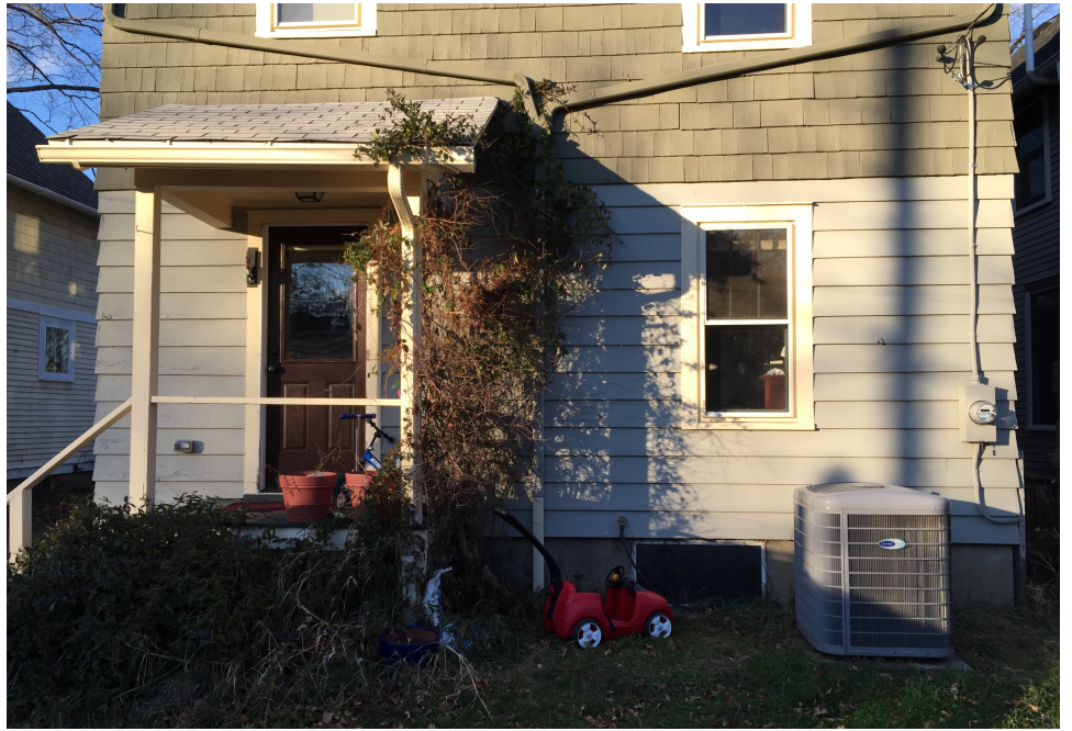
EXISTING REAR ENTRY DECK (PROPOSED MUDROOM LOCATION)
