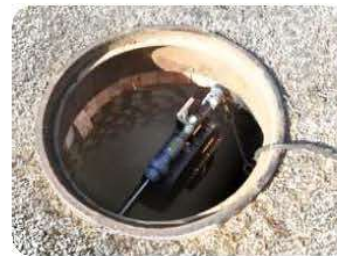
ECHO with tension bar installation
