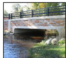
Figure 4: Three-sided box bridge
