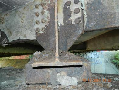
Photo 1: Typical Beam End with Pack Rust
