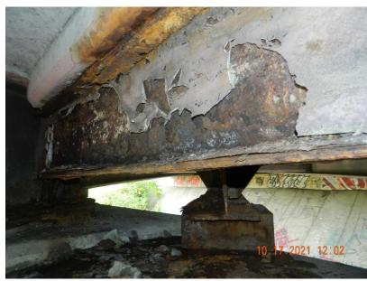
Photo 4: Typical Beam End with Paint System Failure and Section Loss
