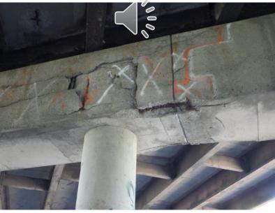
Photo 3: Spalled Pier Cap with Exposed Rebar
