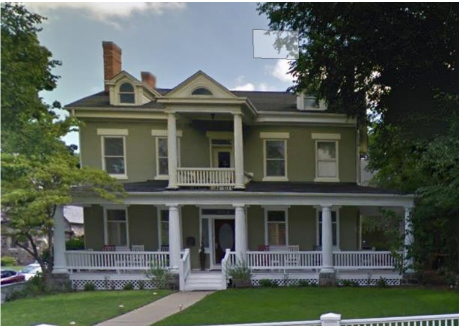
218 N. Division Street (August 2016 Google Street View)
