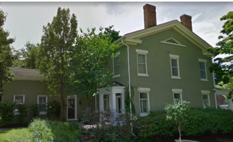
218 N. Division Street (August 2016 Google Street View)
