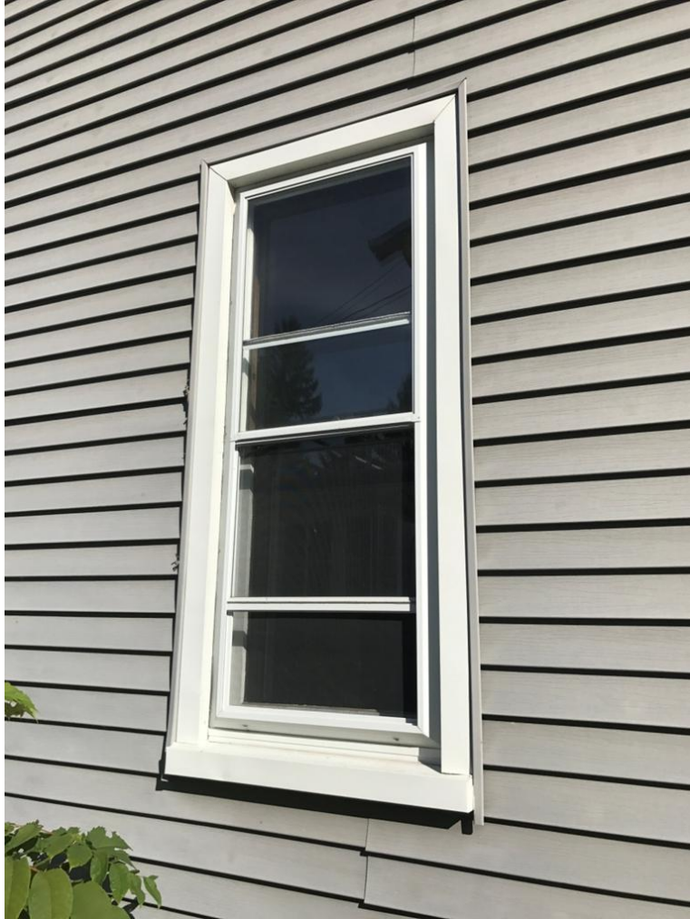
Existing windows with trim boards and aluminum storm windows
