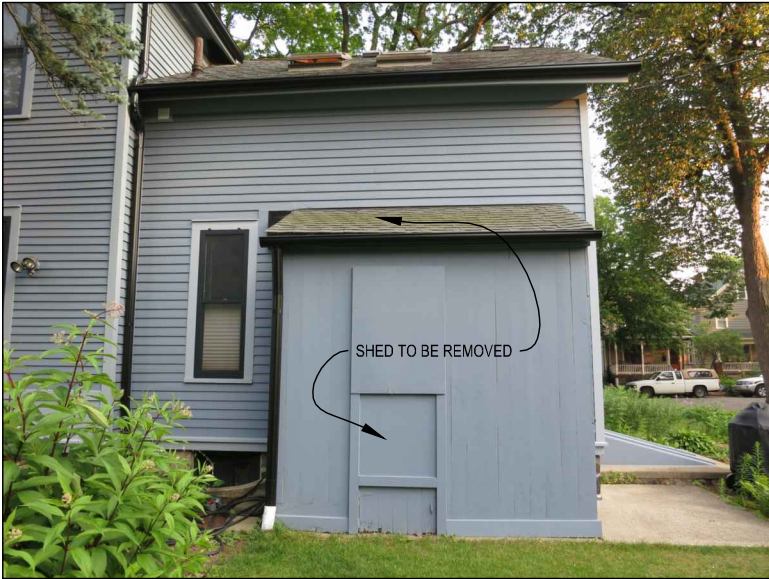
SHED FROM NORTH
