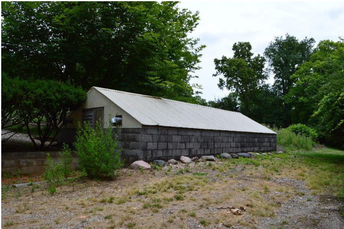
Looking northeast at coldhouse, July 2017
