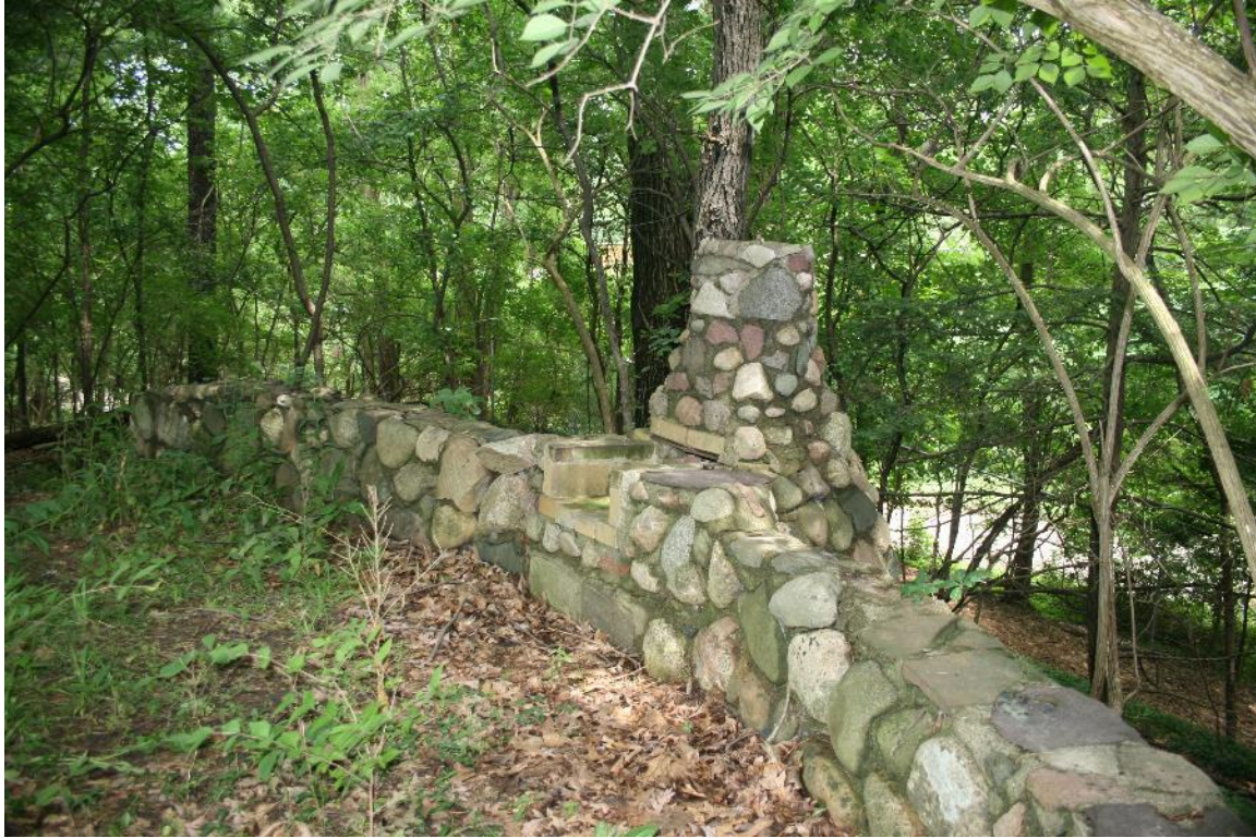
Fireplace built into east wall of wild garden, July 2017
