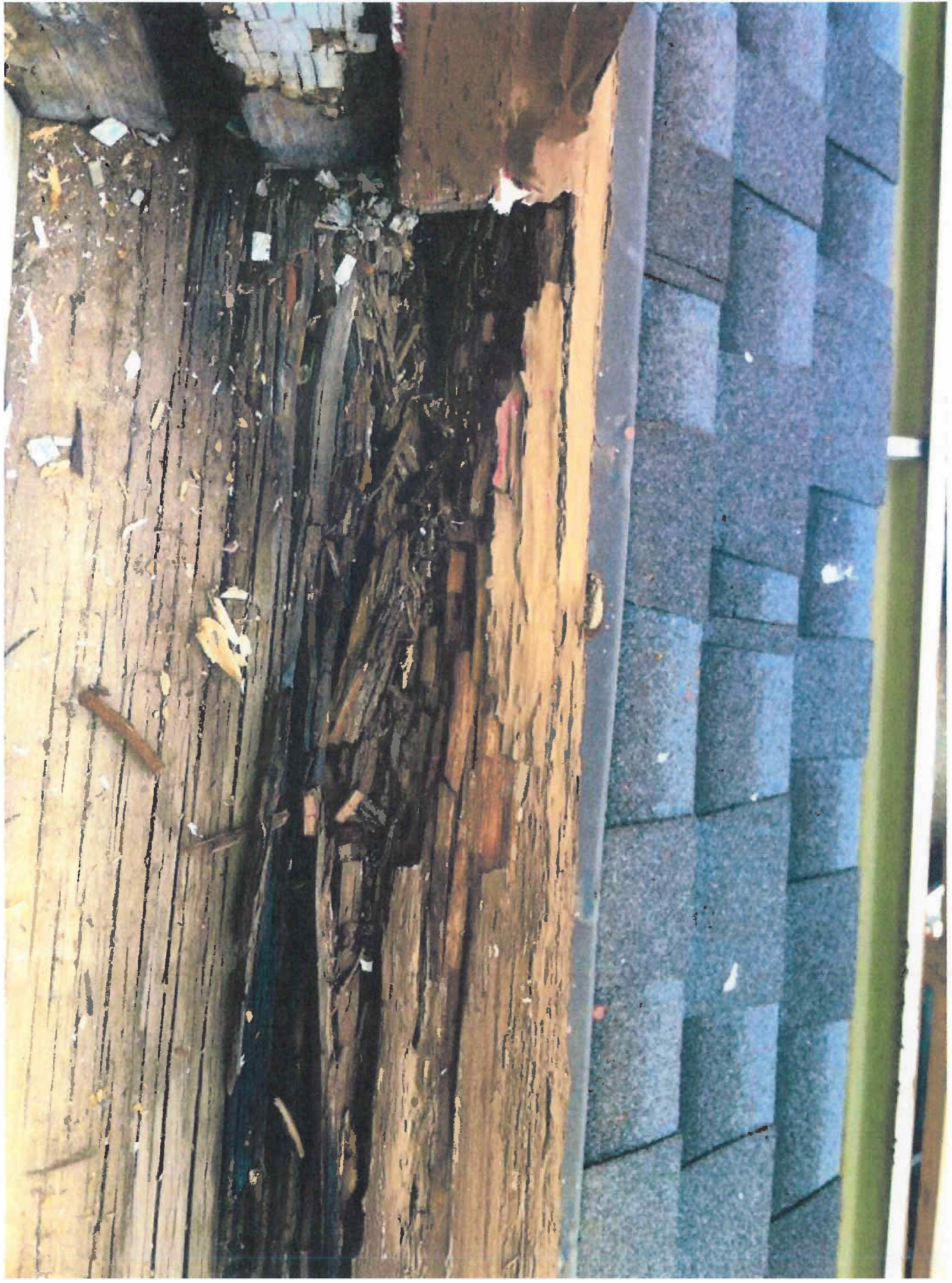
S-1 (South View) condition
