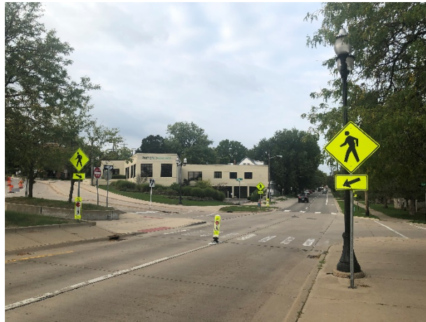
Figure 4 The crosswalk at Broadway and Division includes one in-lane pedestrian sign in the street and one on the island to the left.
