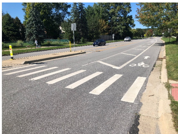
Figure 2 This crosswalk at Green Road and Burbank Road applies high-visibility continental pavement markings.
