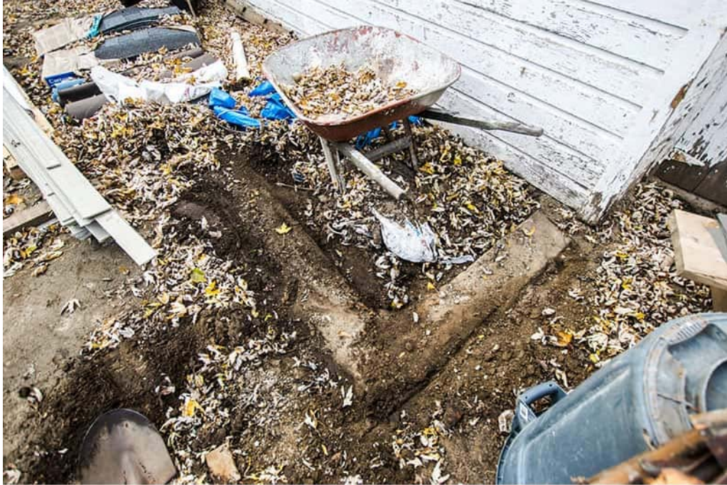
OLD FOUNDATION (south-east corner - matches size in 1947 aerial)
