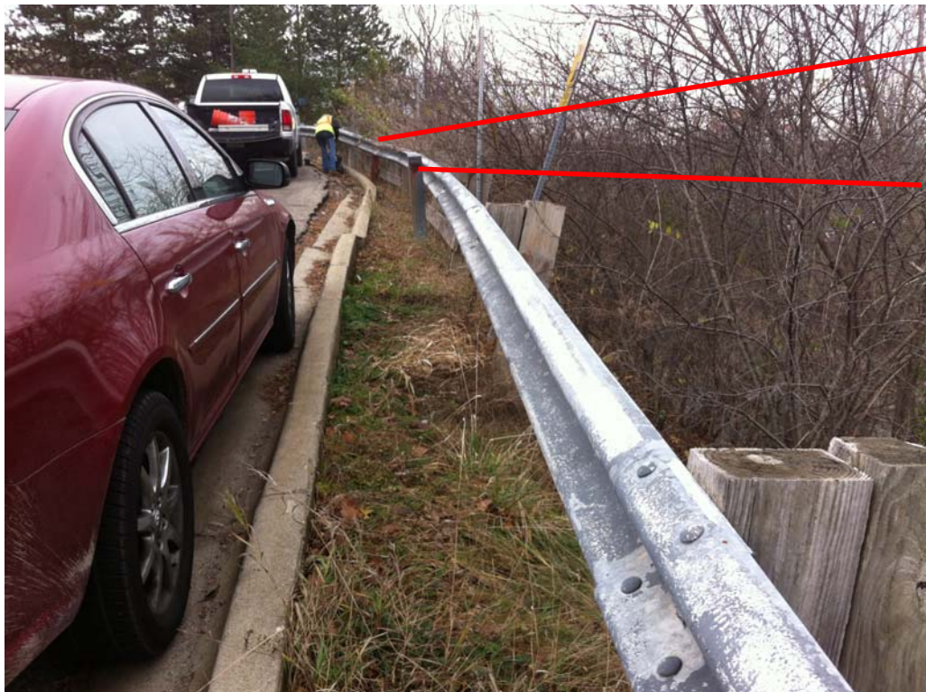
2015 Looking west, toward inclinometers I-1 and I-2
