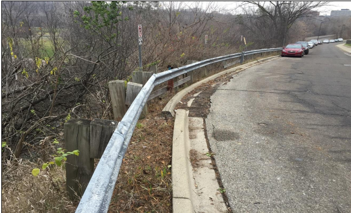
PHOTO NO. 2B - December 12, 2015: Looking east along Nichols Drive from a similar vantage point as PHOTO NO. 2A.
