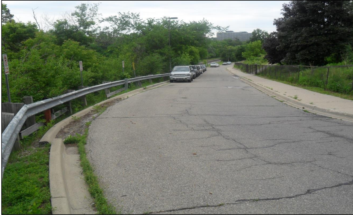
PHOTO NO. 2A - June 11, 2010: Looking east along Nichols Drive.
