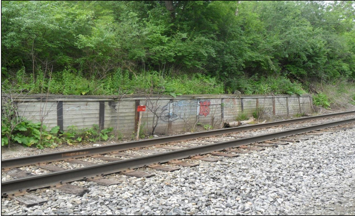
PHOTO NO. 4A – June 11, 2010: Looking at the soldier pile retaining wall at the toe of the slope on the south side of the railroad line.
