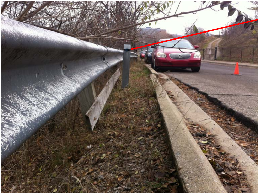
2015 Looking east, toward inclinometer I-2
